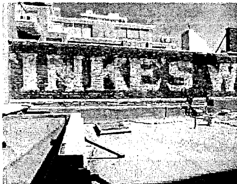
Roof, looking north
