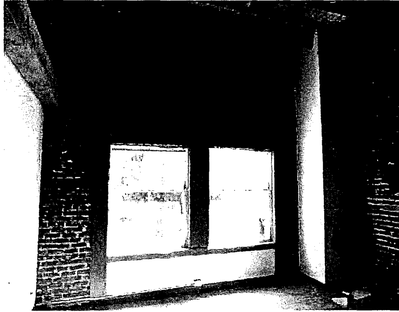
Interior of Montgomery Street 2 nd Floor windows
