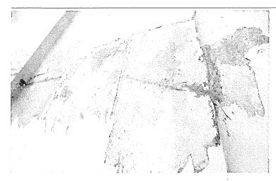
Figure 20. Peeling coating along the north elevation. (Photograph provided by RLJC, April 2015.)
