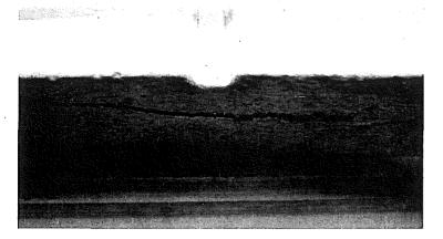
**Figure 17.** Cracked concrete above window at the fifth floor along the north elevation. (Photograph provided by RLJC, April 2015.)
