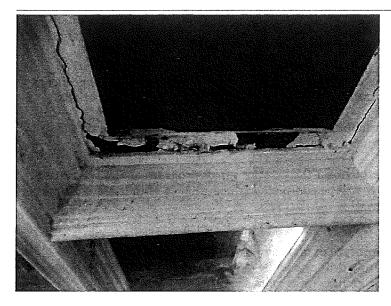
**Figure 22.** Peeling paint and corrosion at ground floor window. (Photograph by Garavaglia Architecture, Inc., April 2015.)
