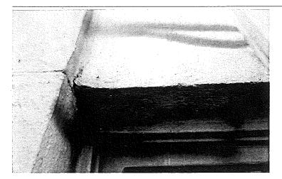
**Figure 18.** Cracked concrete above window at the seventh floor along the north elevation. (Photograph provided by RLJC, April 2015.)
