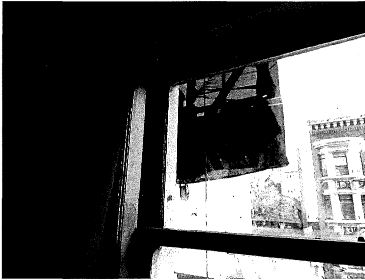
Figure 10. Overview of typical wood double-hung window unit along the north elevation. (Photograph by Garavaglia Architecture, Inc., April 2015.)
