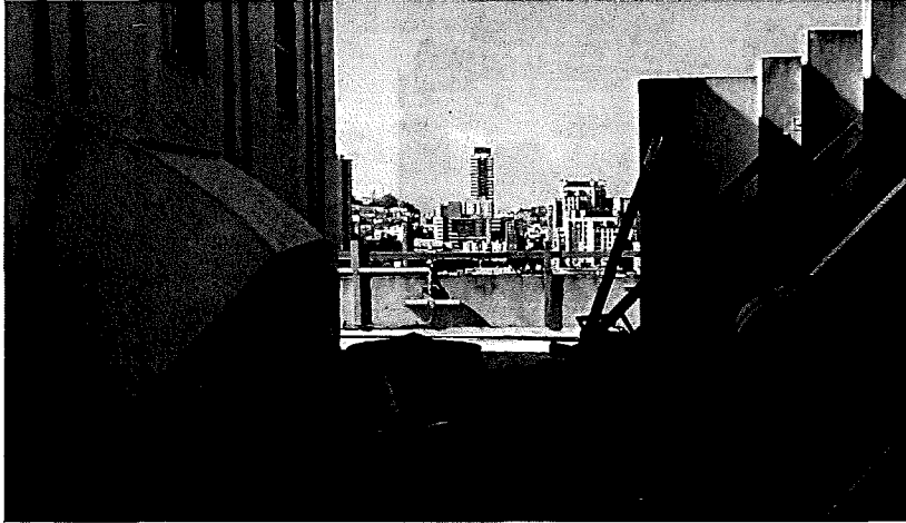
Figure 14. Overview of main roof level, showing mechanical equipment. (Photograph provided by RLJC, April 2015.)
