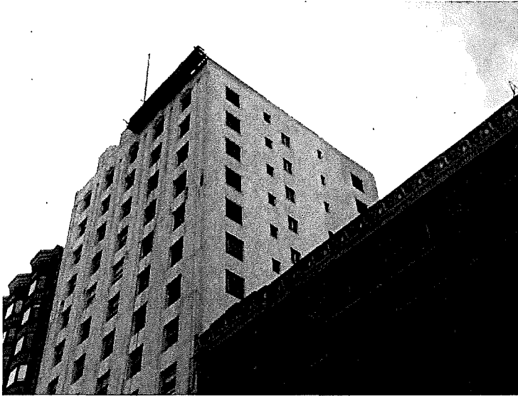
Figure 12. Overview of north and east elevations. (Photograph by Garavaglia Architecture, Inc., April 2015.)
