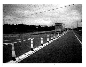
vertical soft-hit posts have been installed in San Francisco such as Market Street, the soft-hit posts are frequently flattened, missing or damaged.
