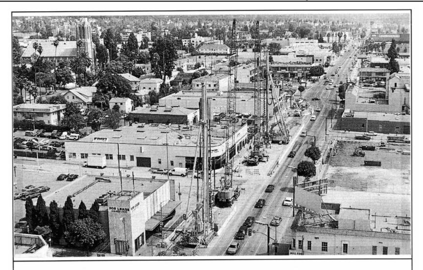
Figure 5.20-1: Soil Cement Wall Augers In Use
