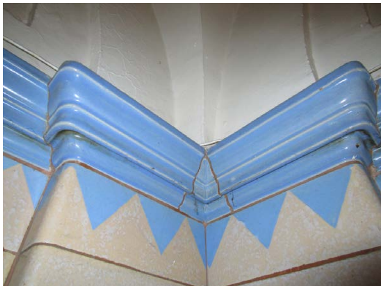
Detail of tile work in entry vestibule
