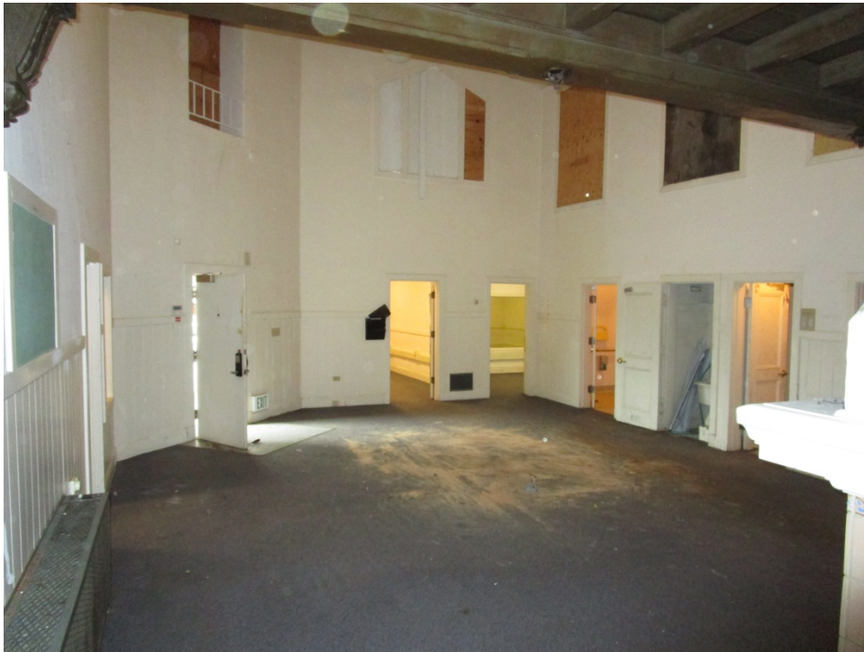
Lobby, view north; note metal railing in punched window opening at second story.
