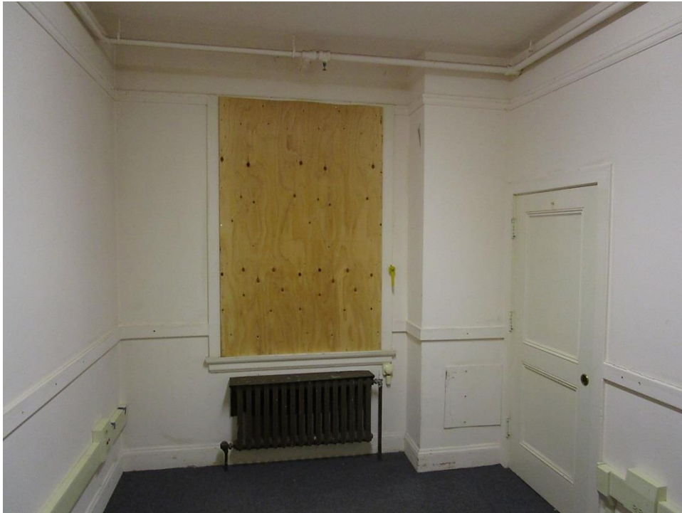
Typical examination room finishes.
