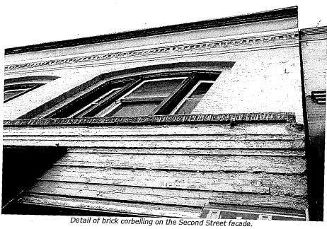
There appear to be several areas of repairs made to the exterior brickwork over time. This includes somewhat crudely executed stucco patching of the corbelled beltcourse separating the first and second stories, as well as patched repair of the dentils below the cornice.
