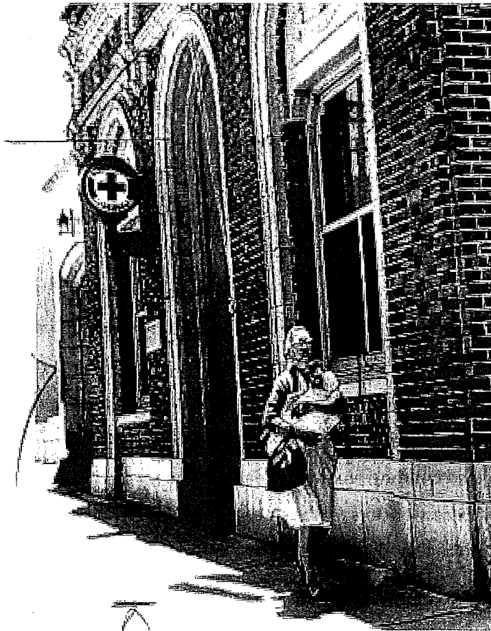
Alemany Emergency Hospital & Health Center, Onondaga and Alemany Boulevard, 1962. San Francisco History Center, San Francisco Public Library. [Note the "Emergency Hospital" sign at entrance.]
