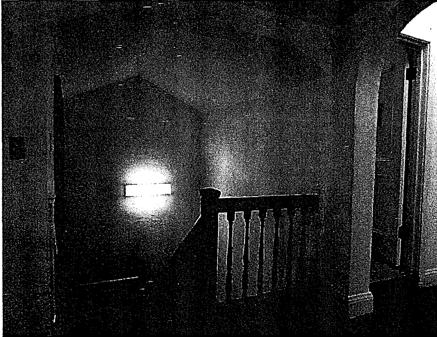
View of stair landing at second floor; note turned wood balusters, vertical board wainscot at staircase, and vaulted ceiling.
