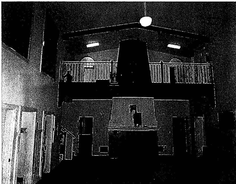
Lobby, view south; note double height volume, gable ceiling with wood beams, balcony, central fireplace with tapered chimney, metal candle scones and openings flanking fireplace and chimney, and vertical board wainscot with flat board trim throughout
