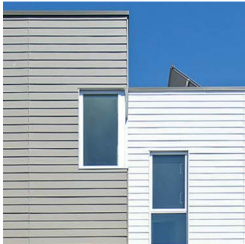
1 LIGHT FIBER CEMENT BOARD HORIZONTAL LAP SIDING
