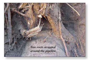
These are the most common examples of how trees planted too near a pipeline can cause damage and leaks that put the community at risk and may possibly disrupt service to our customers.
