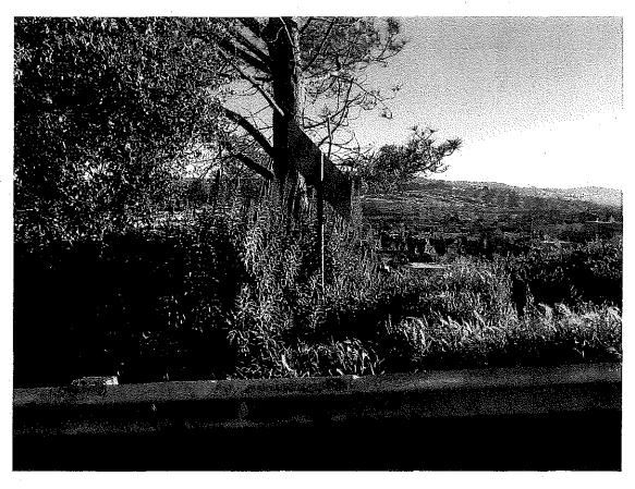
30-foot pine tree growing above PG&E Gas Transmission Pipeline 109 at Bernal Heights Blvd. - in violation of PG&E's threatening the pipelines protective coating.
