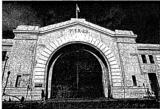
Reopen historic bulkhead and return to economic use
