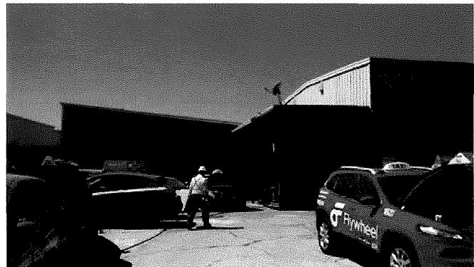
View south of the one-story storage addition.
