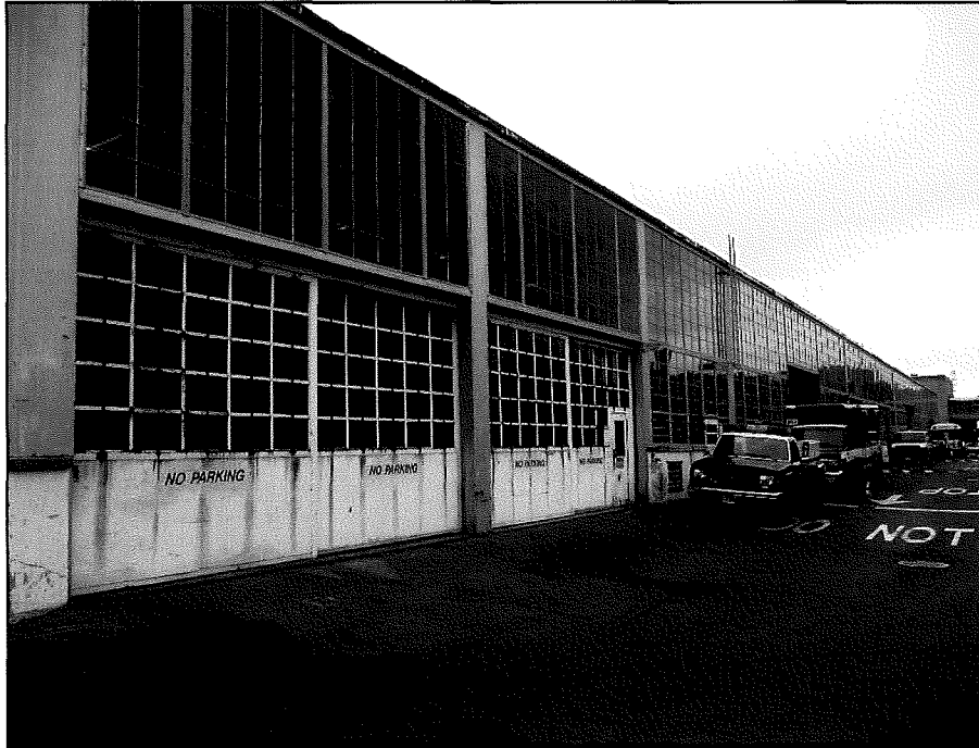
Photograph 6. Building B, camera facing northeast, August 20, 2014.
