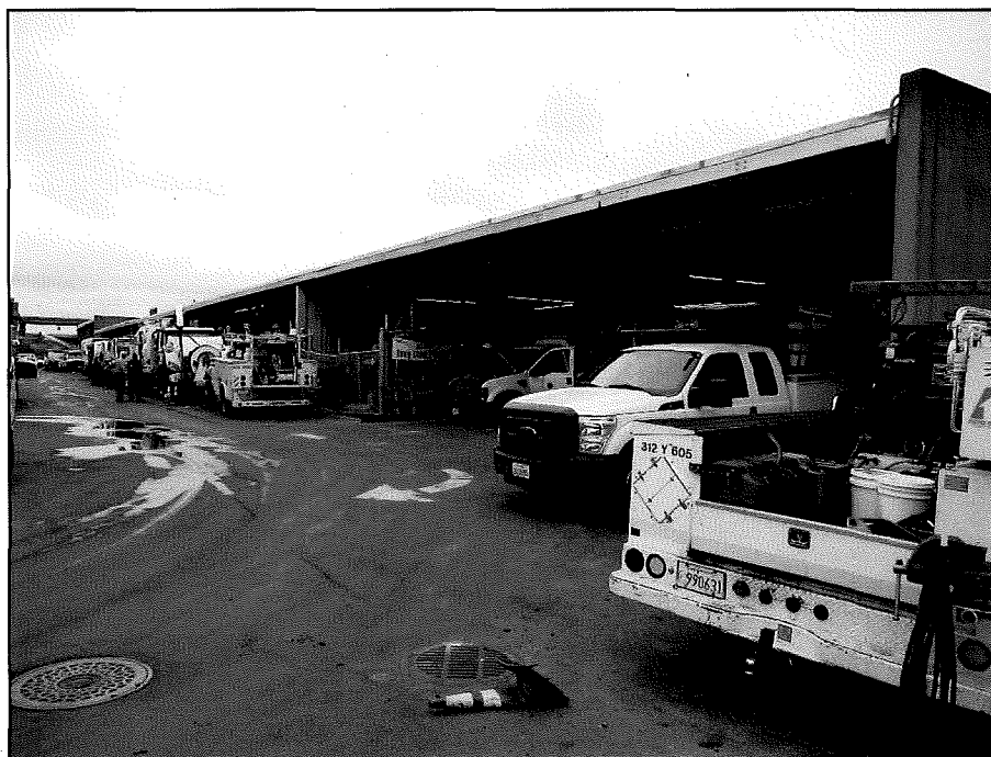
Photograph 9. Building C, camera facing northwest, August 20, 2014.
