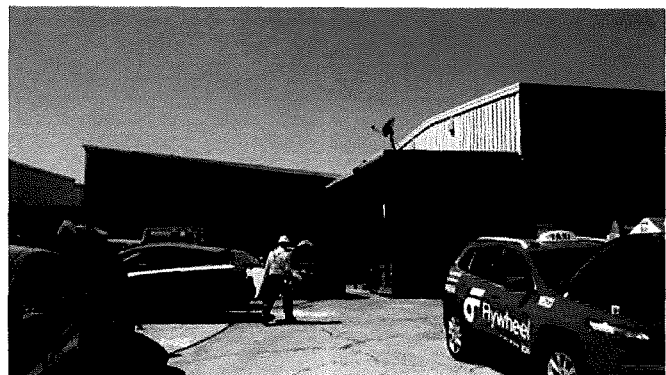
View south of the one-story storage addition.
