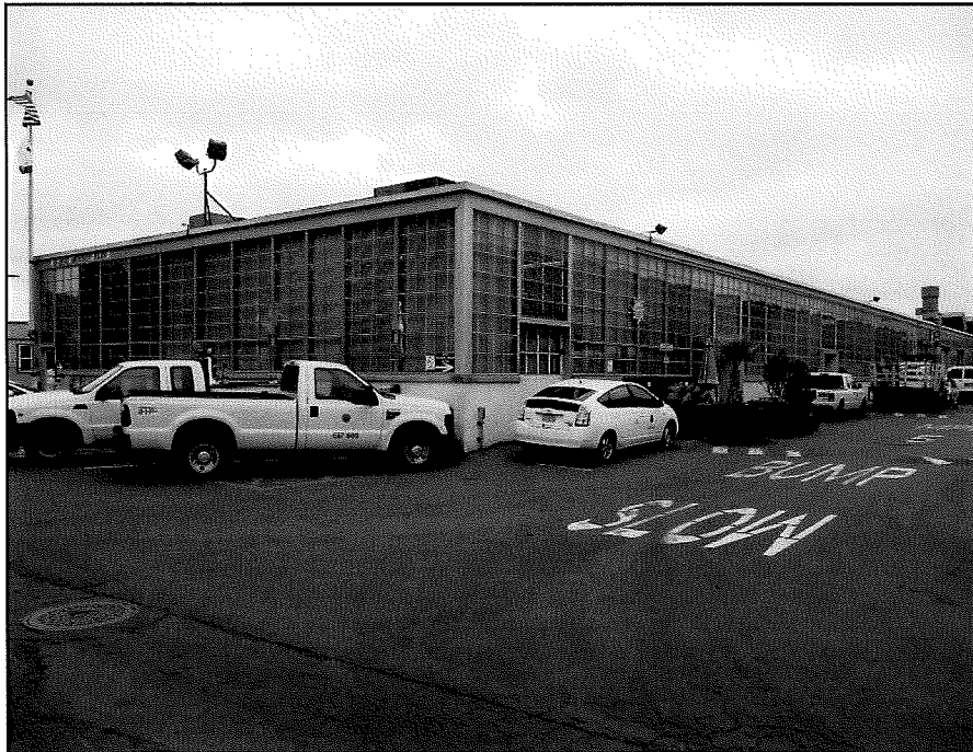
Photograph 2. Building A, camera facing west, August 20, 2014.
