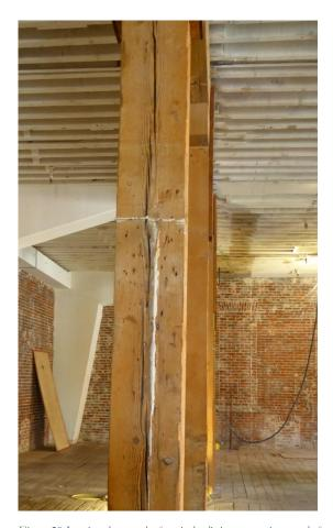
Figure 59 Interior photograph of vertical splitting present in several of the structural timber columns on the ground floor (photography taken on 04/05/2017).
