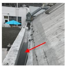
Photo 12: Ponding observed in perimeter drainage trough.
