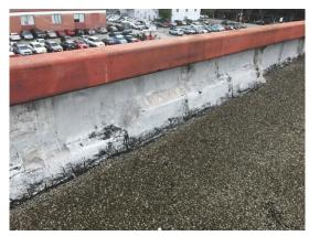
Photo 18: Roof sheet extends up brick parapet.
