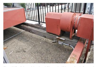
Figure 135 Detail photograph from the roof. Note use of steel I-beams and nominally cut wood to elevate and support HVAC (photograph taken on 04/05/2017).
