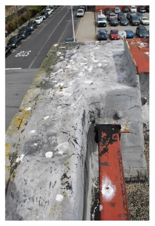
Figure 51 Photograph of the northeast corner and horizontal surface on parapet. Note hiological colonization, corrosion, atmospheric pollution, and animal deposits (photography taken on 04/04/2017).
