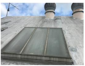
Photo 13: Skylight through steep slope roofing.
