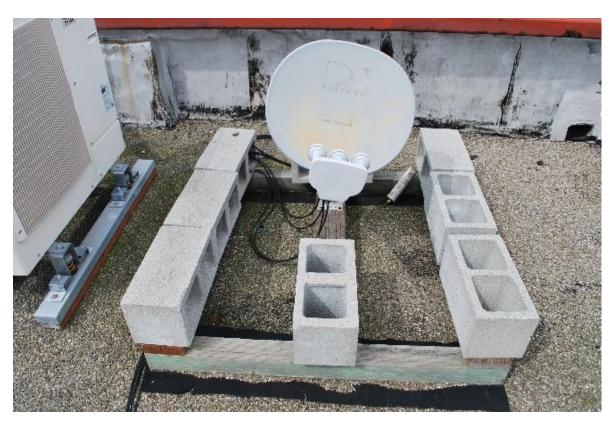
Figure 136 Detail of satellite dish installation. Note use of cinderblocks to weigh down nominally cut wood (cinderblocks are not anchored to the roof). Photograph was taken on 04/05/2017.
