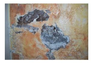
Figure 75 Detail photograph of north foundation condition. Note lost finish, exposed stone, and extensive efflorescence (photography taken on 04/04/2017).
