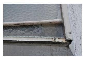
Figure 48 Detail photograph of chicken-wire glass and delaminated paint film (photography taken on 04/04/2017).
