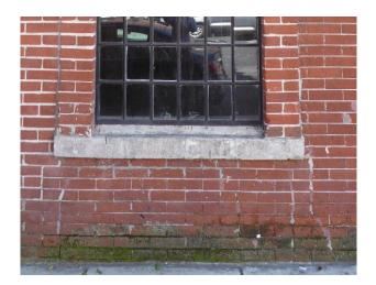
Figure 32 Detail of biological colonization plaguing mortar joints at the bottom courses along Vallejo Street (photography taken on 03/31/2017).
