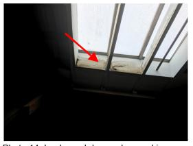
Photo 14: Leaks and decay observed in skylights on the underside.
