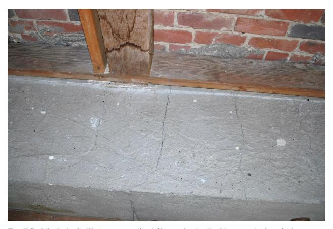
Figure 80 Detail of modern lateral stabilization system (concrete beams). Note severe through-cracking of the cement matrix (photography taken on 04/04/2017).
