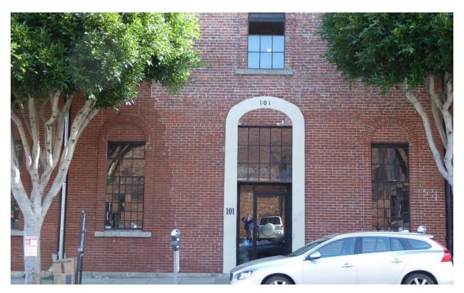
Figure 27 Photograph of 101 Vallejo Street. Note visual seam between historic brick (left) and the brick used in a later restoration campaign (right). Photography was taken on 03/30/2017.
