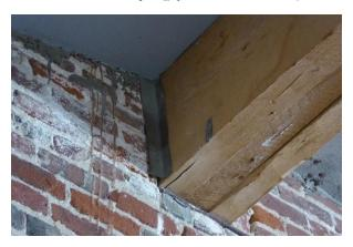
Figure 109 Interior detail of structural timber-to-brick construction. Note the use of steel angles and flashing (photograph taken on 04/10/2017).
