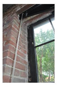
Figure 130 Detail photograph of window hardware on the second floor. Same window as previous two images. This is believed to be the earliest construction type found for the windows (photograph taken on 04/04/2017).
