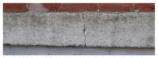
Figure 33 Detail of Vallejo Street water table. Note fragmentation of granite via through-cracking, Also note hairline cracking condition found in cement plaster stucco at foundation (photography taken on 03/31/2017).
