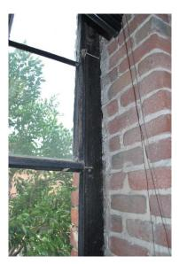
Figure 129 Detail photograph of window hardware on the second floor. Same window as left image. This is believed to be the earliest construction type found for the windows (photograph taken on 04/04/2017).
