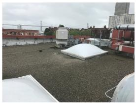
Photo 19: Several pieces of equipment and skylights on low slope roof.
