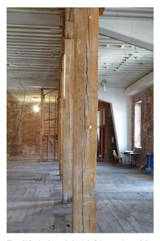
Figure 58 Interior photograph of vertical splitting present in several of the structural timber columns on the ground floor (photography taken on 04/10/2017).
