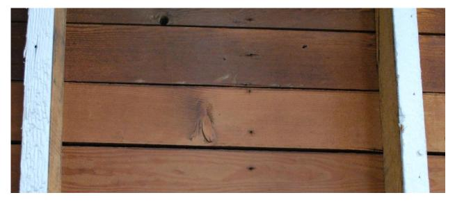
Figure 132 Detail of roof construction on the east wall. Only roof wall found to have wood instead of corrugated metal (photograph taken on 04/05/2017).
