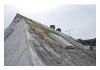
Figure 45 Detail of north facing hip of the roof. Note heavy biological colonization (photography taken on 04/05/2017).
