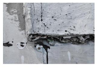
Figure 47 Detail photograph of roof waterproofing construction. Materials include tar, sheet metal, and titanium synthetic underlayment (photography taken on 04/05/2017).
