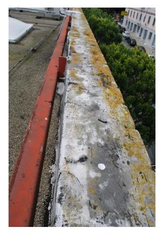
Figure 52 Photograph of horizontal surface on east parapet. Note biological-colonization, corrosion, atmospheric soiling, and minor animal deposits (photography taken on 04/04/2017).
