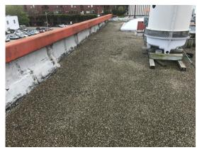
Photo 17: Low slope roof with built-up roof (BUR) and gravel topping.
