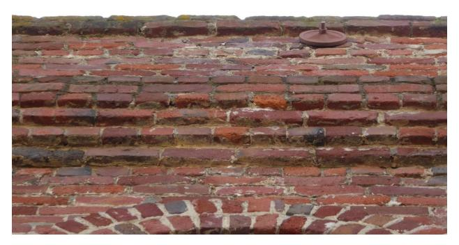
Figure 98 Detail view of corbeled cornice and parapet wall along Vallejo Street (photograph taken on 03/30/2017).
