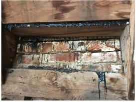
Photo 6: Roofing tar leaking through slats in wood sheathing.
