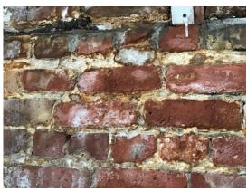
Photo 9: Deterioration in mortar joints of brick wall below gutter.
