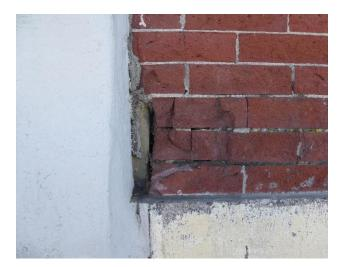
Figure 15 Detail of water table, door surround, and brick facade intersection. Note remaining paint on the watertable granite (photography taken on 03/31/2017).
