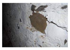
Figure 76 Detail photograph of south foundation wall. Note delamination of finish, spalling and disaggregation of fieldstone (photography taken on 04/04/2017).
