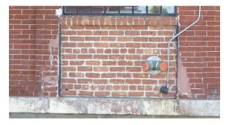
Figure 11 Detail of mismatched brick in-fill under window opening along Front Street (photography taken on 03/30/2017).
