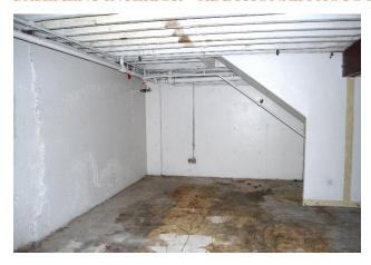
Figure 115 Interior photograph at the basement. Note seam between concrete and stone foundations (left). Photograph was taken on 04/04/2017.
