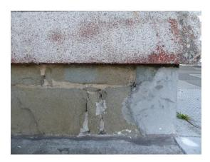
Figure 6 Detail of foundation condition. Note Portland cement mortar replacement and patching (photograph taken on 03/31/2017).
