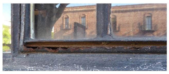
Figure 26 Detail of localized corrosion and window sash failure. Instances are few, however, need repair/rehabilitation (photography taken on 03/31/2017).
