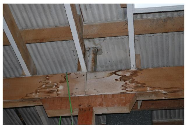
Figure 82 Detail of roof to beam construction. Note water staining and efflorescence on wooden members (photography taken on 04/04/2017).
