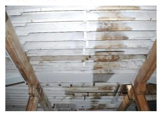
Figure 103 Photograph of ground floor ceiling joists. Note ghosts from old HVAC and water staining (photograph taken on 04/04/2017).
