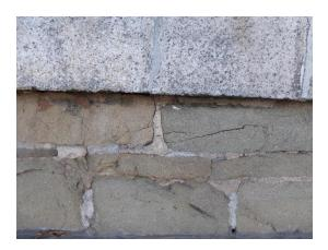
Figure 5 Detail view of foundation stone condition. Note cracking, fragmentation, insipient spalling, and failed mortar joints (photograph taken on 03/31/2017).
