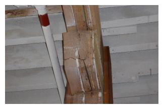
Figure 108 Interior detail of structural timber construction. Note split in capital (photograph taken on 04/10/2017).
