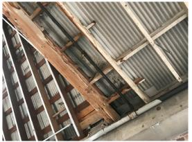
Photo 20: Leak at Northeast corner of low slope roof where it intersects with steep slope roof.
