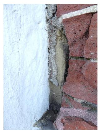
Figure 92 Photograph of entrance threshold at Front Street elevation. Note sandstone substrate (photograph taken on 03/31/2017).
