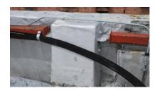
Figure 43 Detail of extant hollow-steel-column to concrete pier construction (photography taken on 04/05/2017).
