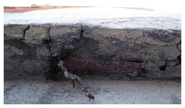
Figure 99 Detail view of cement stucco over brick construction along the V allejo S treet entrances (western two entrances). Photo taken from the foundation and looking up towards the cornice (photograph taken on 03/30/2017).
