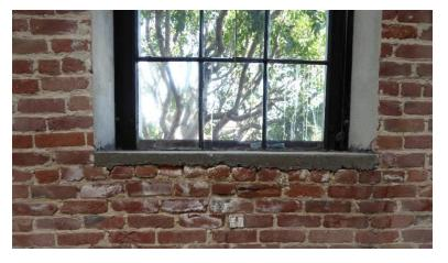
Figure 85 Detail photograph of southernmost window on the east wall. Note occurrence of efflorescence and eroded mortar (photography taken on 04/04/2017).
