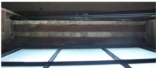
Figure 111 Detail view of lintel construction at window openings. Note cracking of parging coat typical (photograph taken on 04/05/2017).
