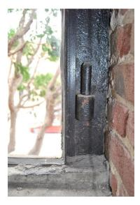
Figure 128 Detail photograph of window bardware on the second floor. Four of these are used in each window, two lower and two upper. This is believed to be the earliest construction type found for the windows (photograph taken on 04/04/2017).
