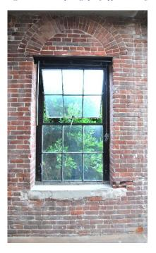
Figure 125 Interior photograph of typical deterioration around window opening (photograph taken on 04/04/2017).
