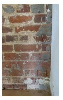
Figure 63 Detail of Portland cement patch and subsequent crack as a result (photography taken on 04/10/2017).
