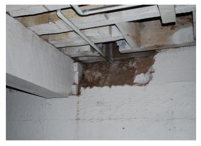
Figure 78 Detail photograph of eroded foundation on the east foundation wall (photography taken on 04/04/2017).
