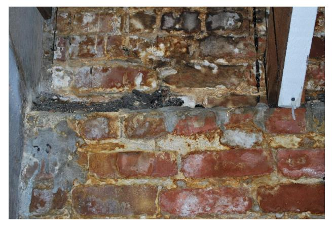
Figure 83 Detail photograph of interior upper brick courses, just below roofline. Note extensive efflorescence and discoloration. The corrosion colored staining is a leaching of ferruginous mineral inclusions innate in the brick and/or mortar (photography taken on 04/04/2017).
