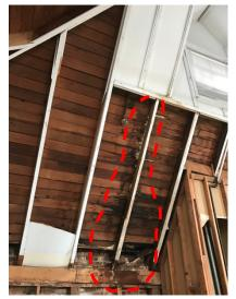
Photo 7: Severe decay in roof framing members.
