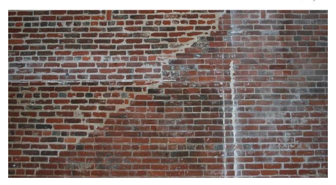
Figure 67 Photograph of south wall at the ground level. Note distinctively different eras of brick and mortar (photography taken on 04/04/2017).
