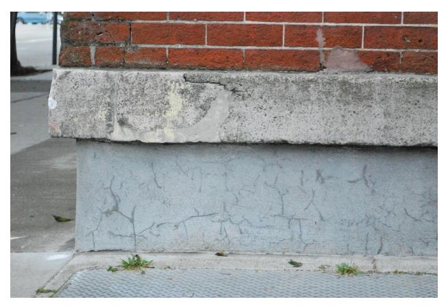
Figure 18 Detail of parging mixture used in the foundation of the Vallejo Street elevation. Note hairline cracking of parging mixture (photography taken on 04/04/2017).
