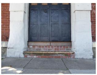
Figure 89 Detail view of entrance bay along Front Street. Note biological activity on brick coursework (photograph taken on 03/30/2017).
