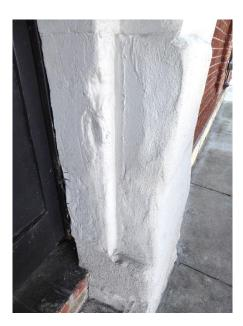
Figure 94 Detail view of cement parging repair on sandstone pilasters (photograph taken on 03/31/2017).
