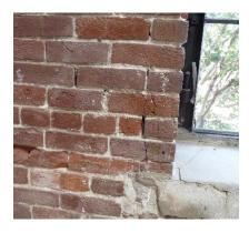
Figure 86 Detail of typical brick condition for deteriorated bricks around window openings (photography taken on 04/04/2017).
