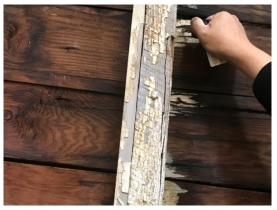
Photo 8: Severe decay in roof framing members.
