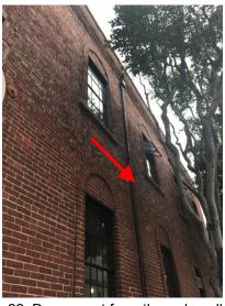
Photo 22: Downspout from through-wall drain.
