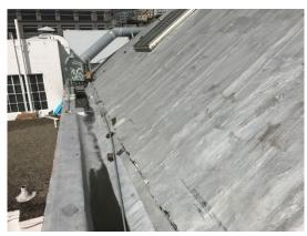
Photo 4: Steep slope roof with aluminum roofing coating.
