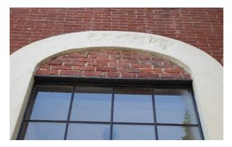
Figure 20 Detail of blind arch at westernmost entrance along Vallejo Street. Note the loss of concrete plaster and the raised metal rebar. Condition is also observed at the 101 Vallejo entrance (photography taken on 03/30/2017).
