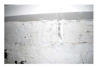
Figure 117 Detail view of south foundation wall. Note irregularly-cut and laid fieldstone (photograph taken on 04/04/2017).
