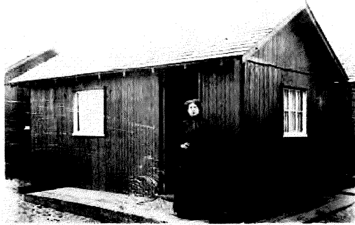
Figure 10. Earthquake shack, 1906. Note exposed rafter tails, wood shingles and round flue (San Francisco History Center, San Francisco Public Library).
