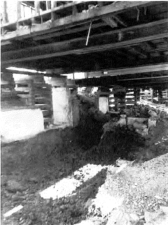
Cottages shored and cribbed during Rehabilitation
