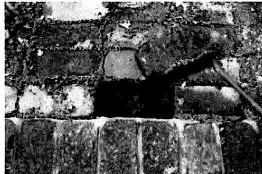
Figure 3: Bedding is a soil/sand mixture
