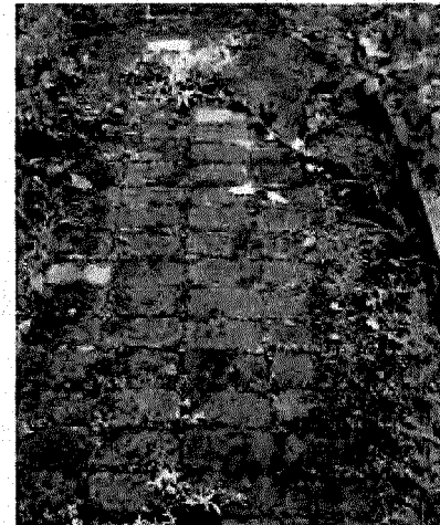
Figure 4: Walkway showing "stacked" coursing and raised brick planter
