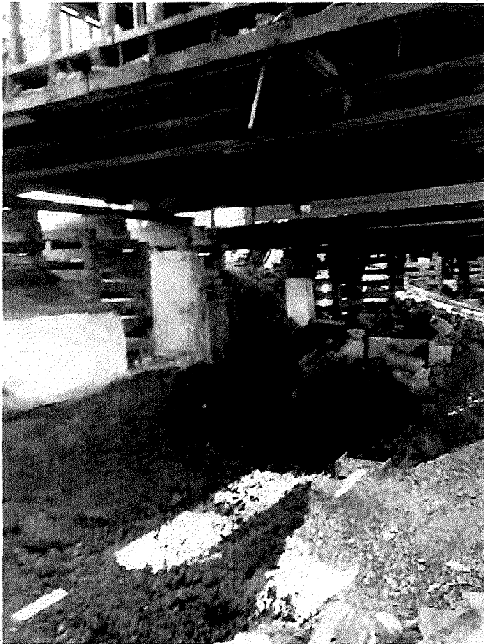
Cottages shored and cribbed during Rehabilitation
