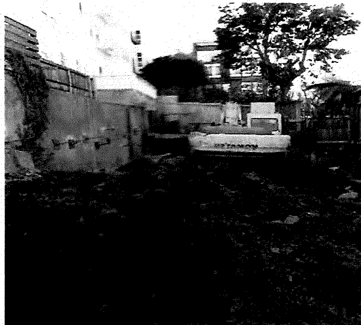
Ties Backs in Consolidated Larkin Retaining Walls
