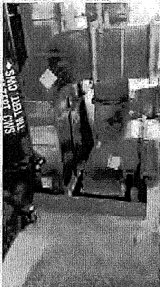
Metal Curb around Dryer Ducting
