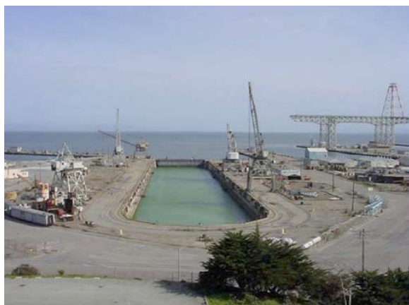
Figure 12. Dry Dock 4, 2008. This was the largest drydock in the world when it was constructed in 1943. Photo: Circa, 2008.
