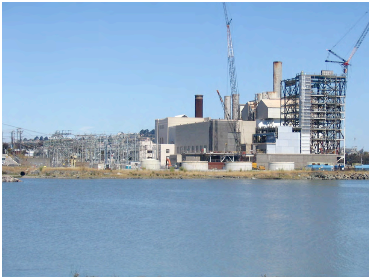
Figure 15. The Hunters Point PG&E plant during deconstruction, July 2007. The entire plant was removed by July 2008. Photo by Circa: Historic Property Development.
