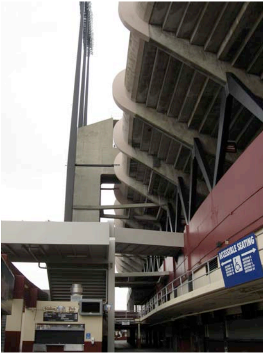
Figure 15. Concrete buttress (in front of light tower) added c.1970 (Mike Gay). (Photo by Circa, 30 January 2010).
