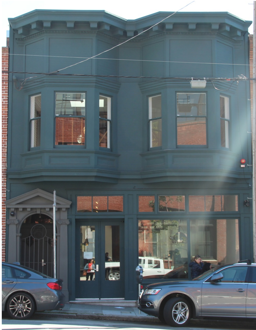
457 BRYANT STREET Pile Drivers, Bridge and Structural Ironworkers Local No. 77 Union Hall
