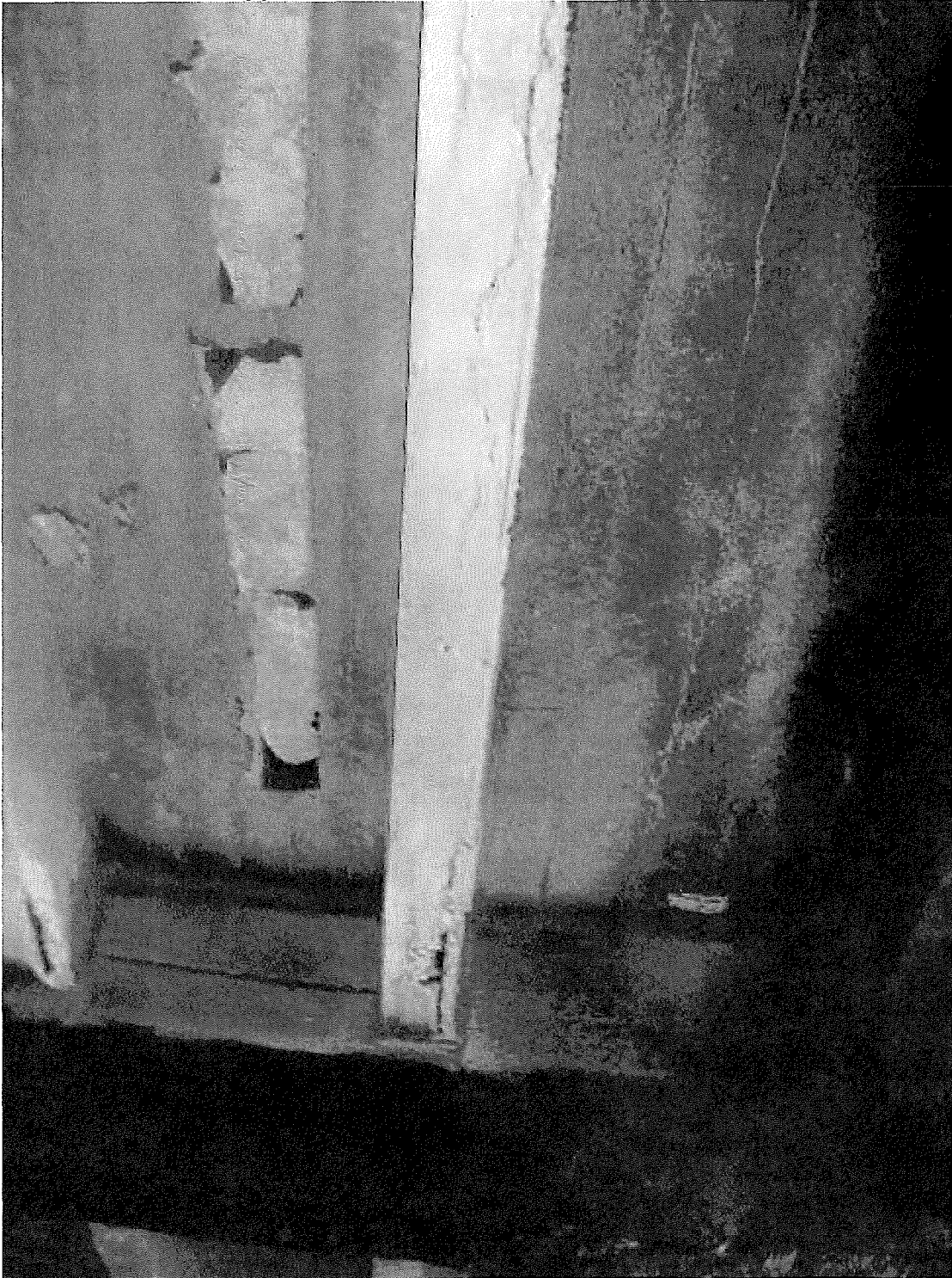
Photo 6. Concrete spalling at slab
