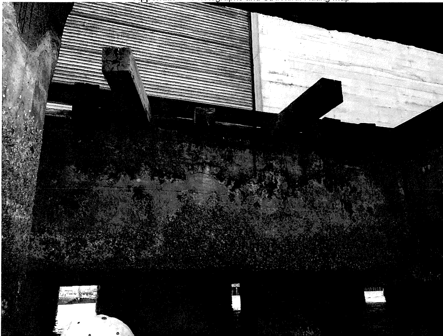
Photo 4. Hole in deck, hanging wood members
