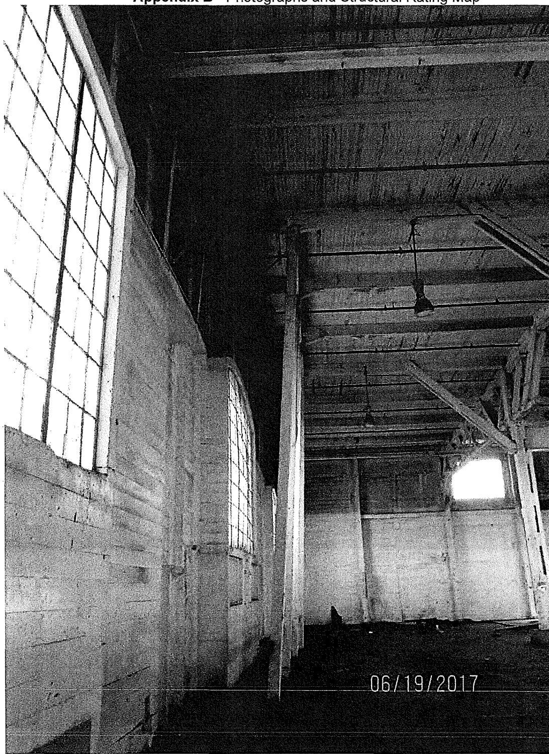
Photo 13. Shoring posts under roof beams near rear wall. Posts are keyed into substructure concrete slab.
