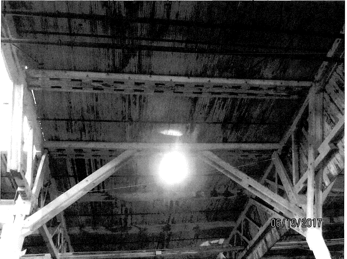
Photo 14. Wood roof beams strengthened in the past.
