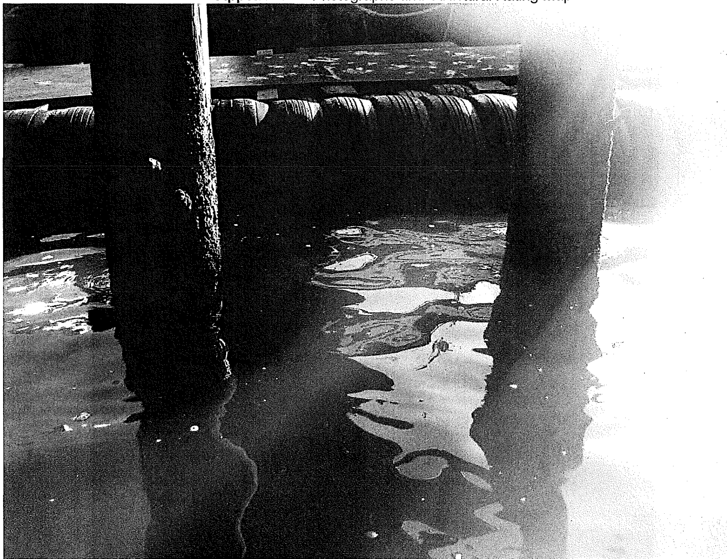
Photo 4. Deteriorated wood piles near metal deck
