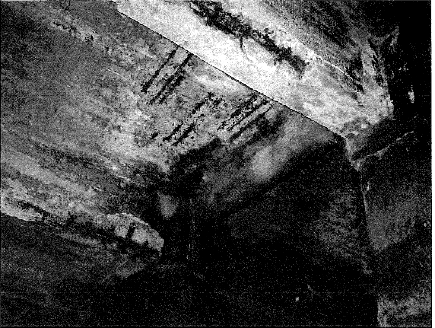
Photo 9. Spalling of concrete beams and slab
