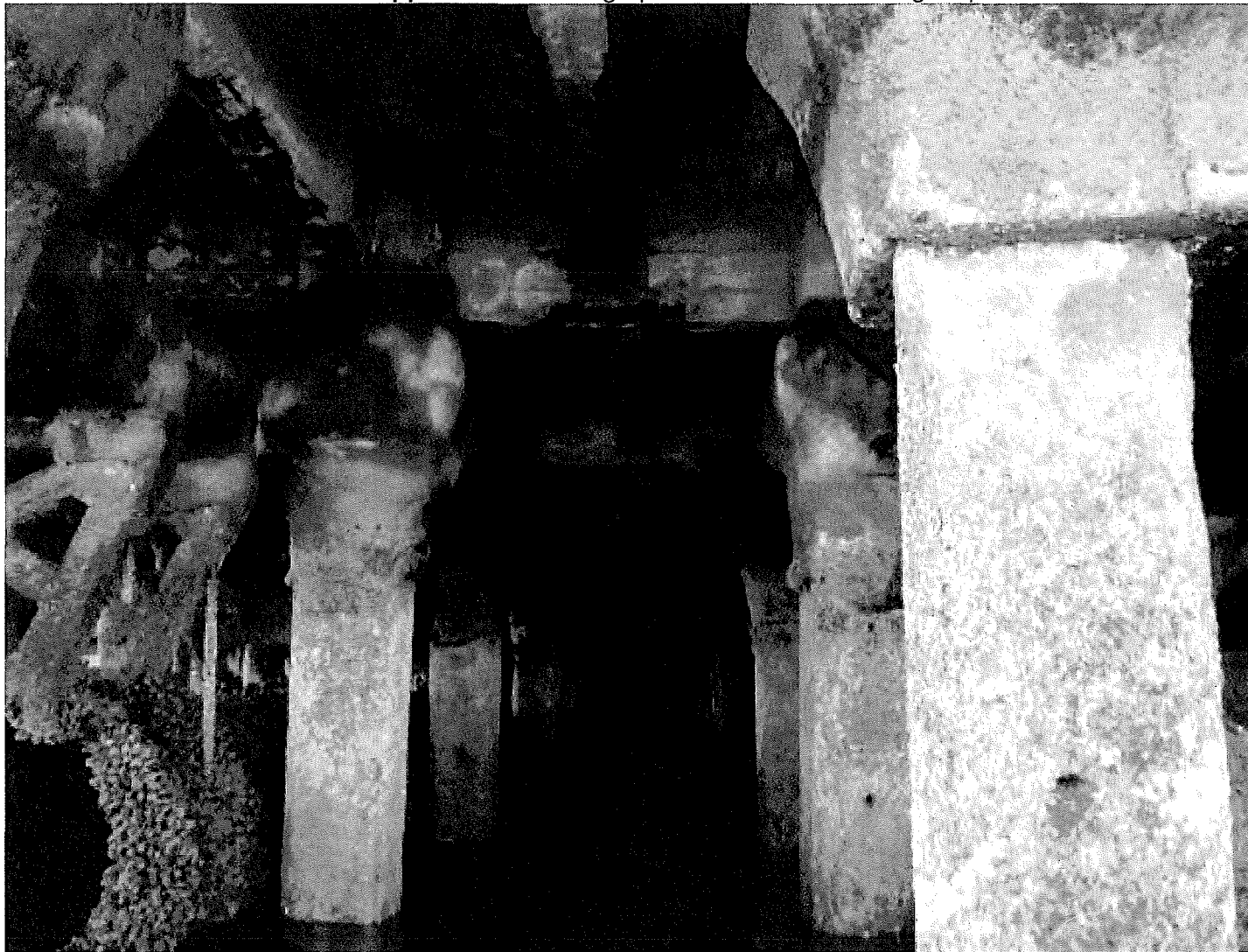
Photo 1. Spalled concrete beams and slabs above the outfalls under the Main Pier
