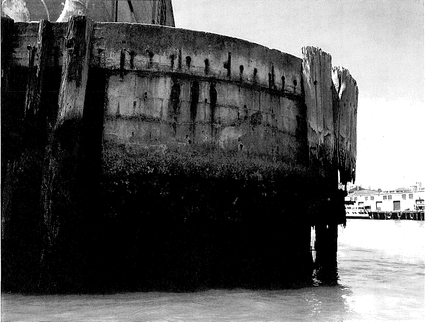
Photo 3. Deteriorated wood piles at pier corner
