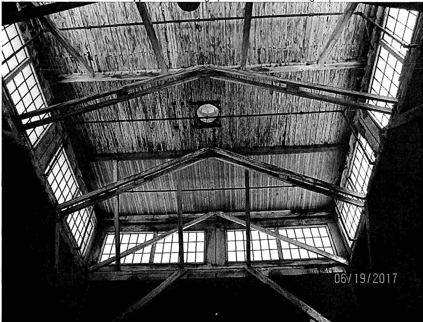
Photo 10. Roof monitor with new beam and 2x4 sheathing.
