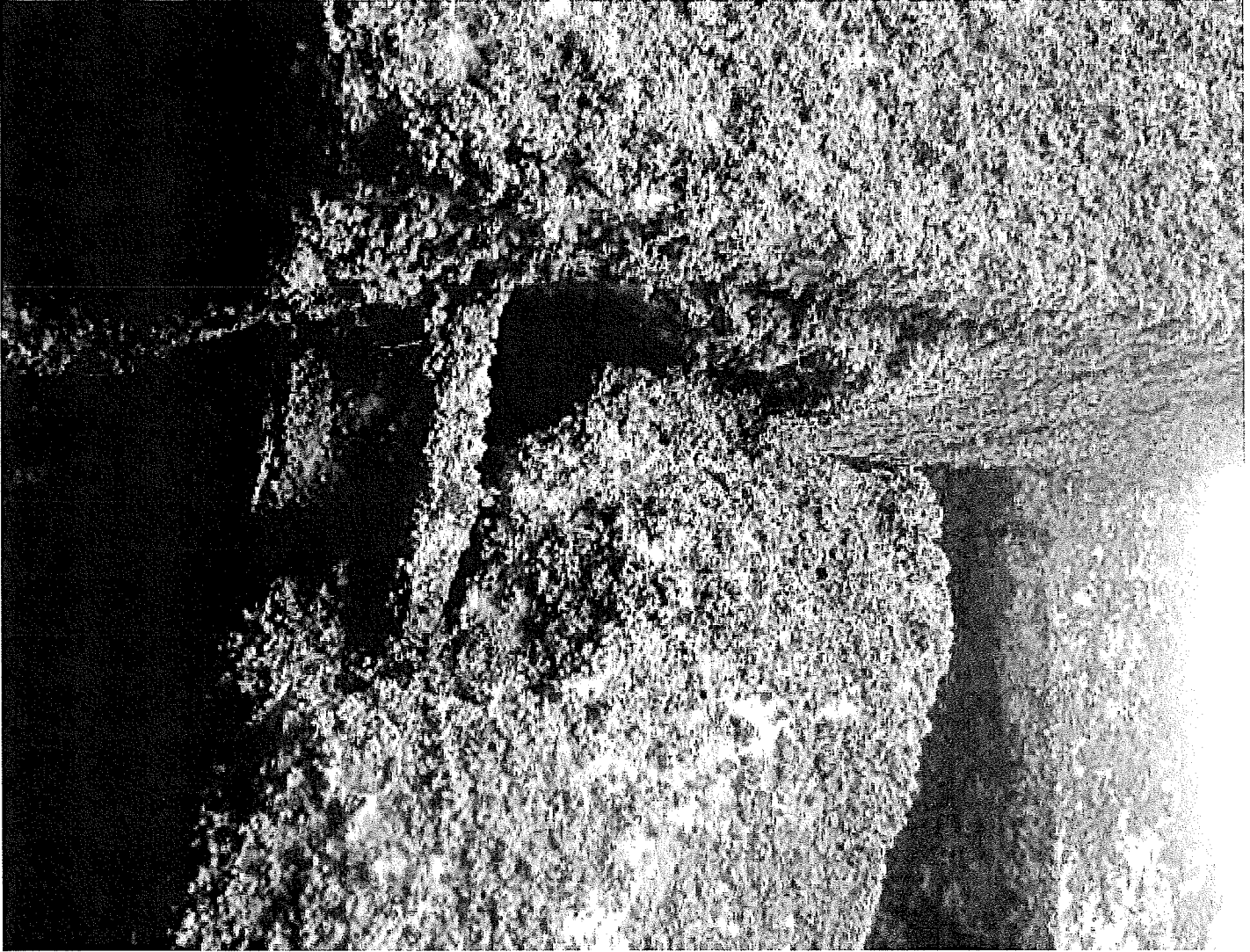
Photo 11. Close up of broken batter pile
