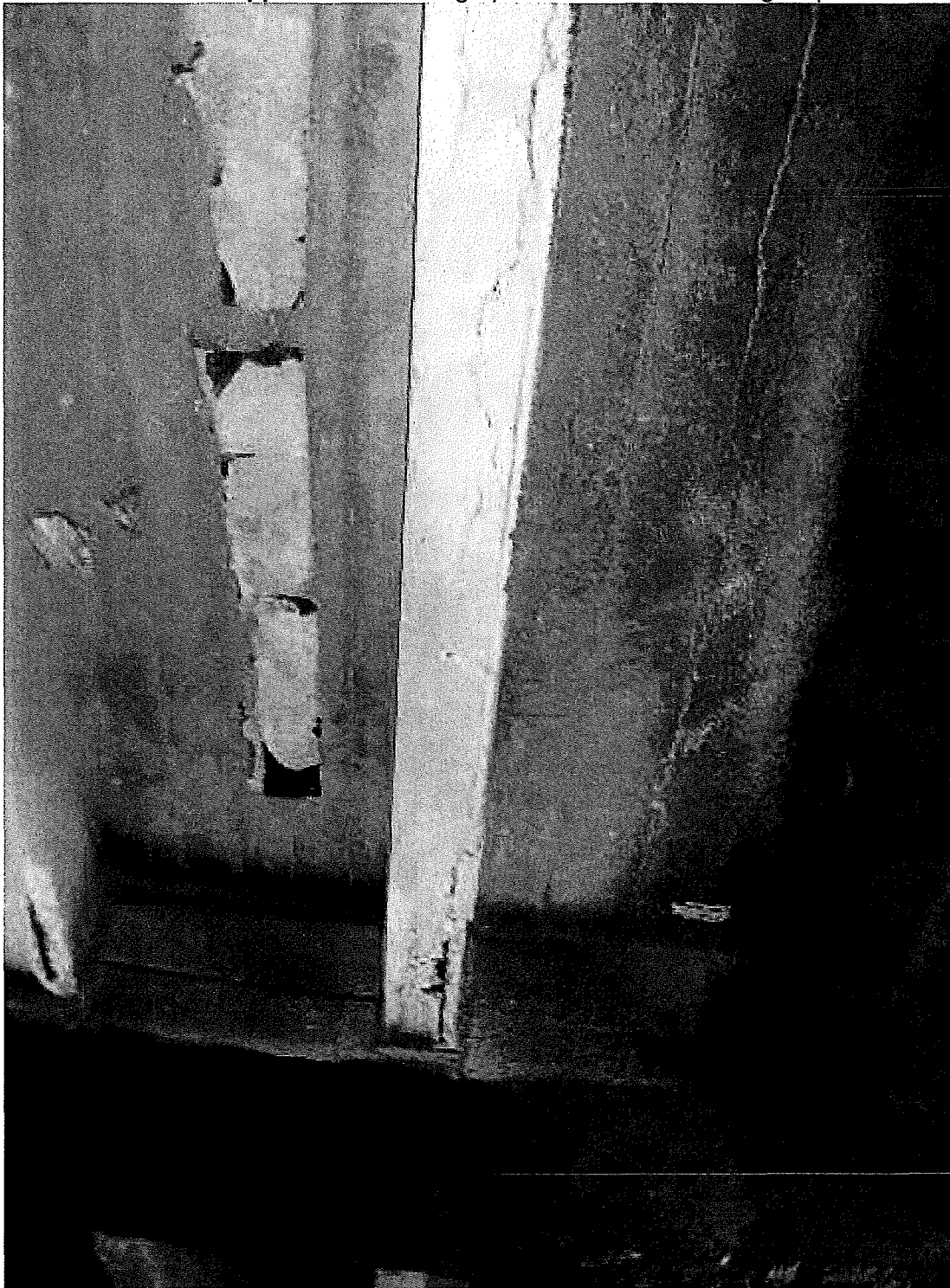
Photo 6. Concrete spalling at slab
