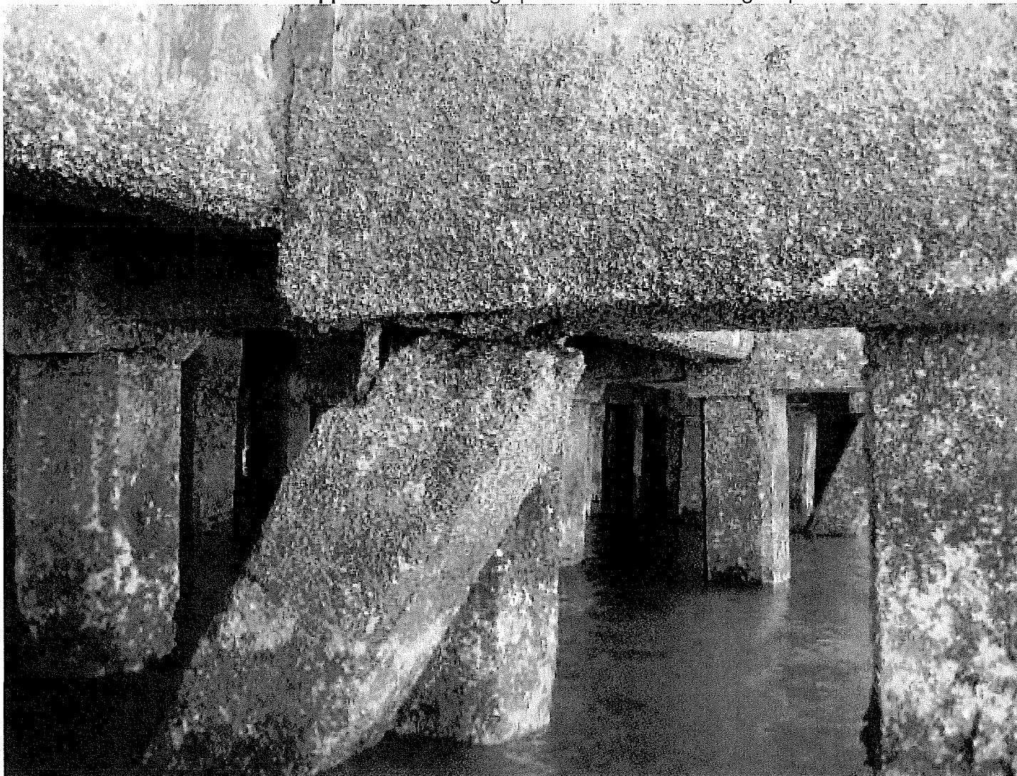
Photo 7. Broken batter pile
