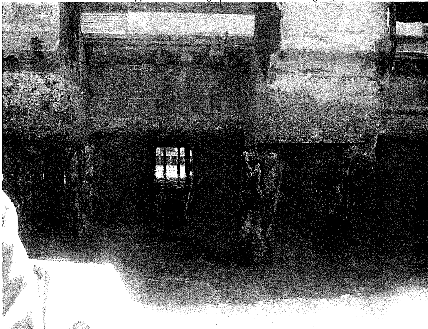
Photo 5. Deteriorated fender piles
