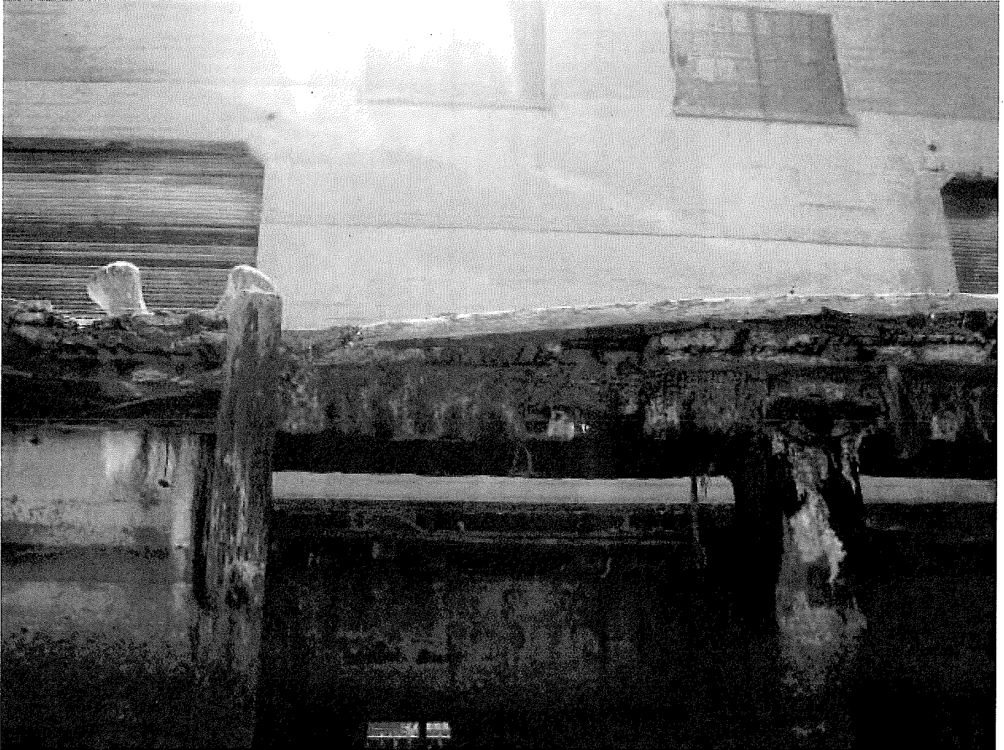
Photo 10. Spalling deck and corroded/exposed rebar
