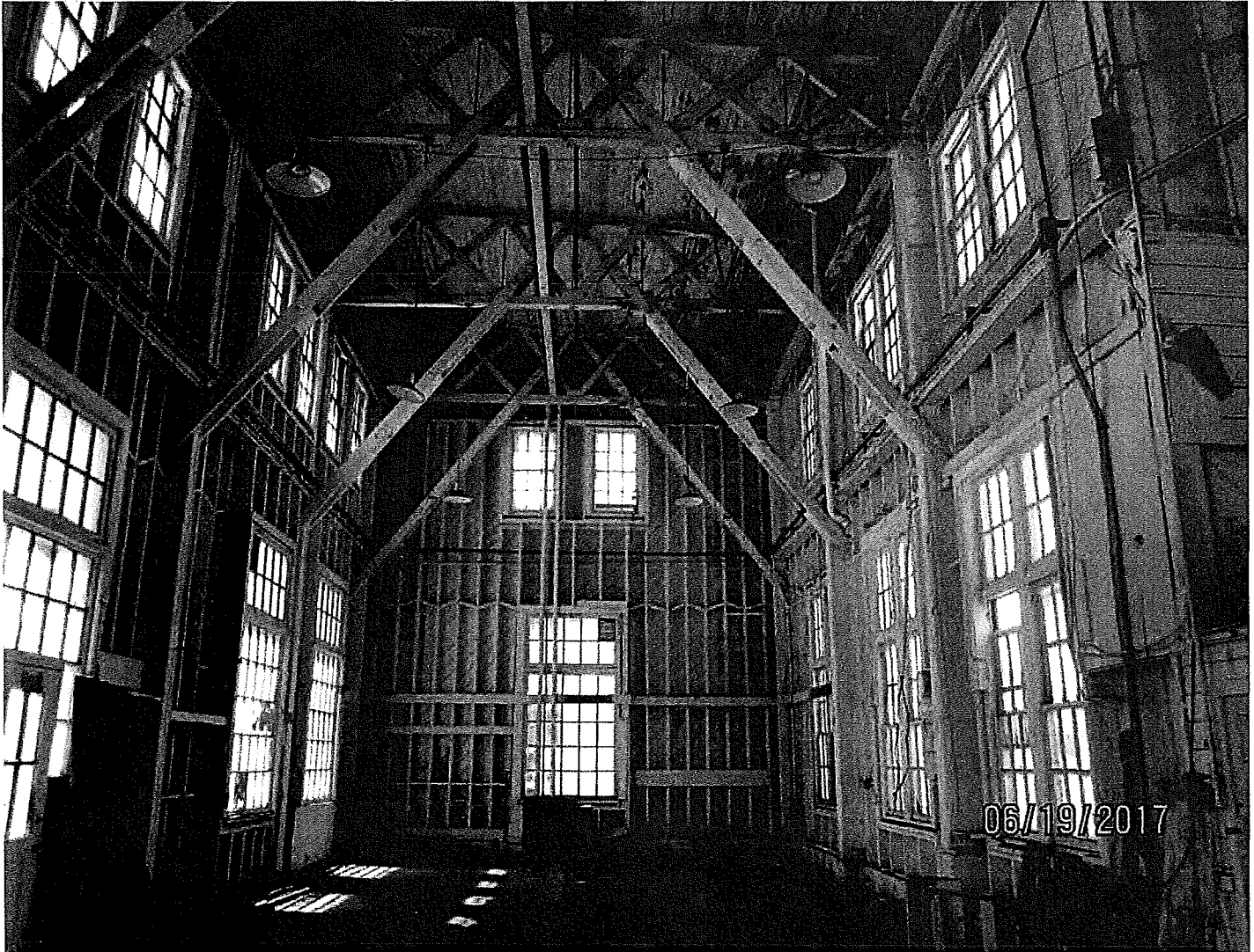
Photo 5. Typical bulkhead framing.
