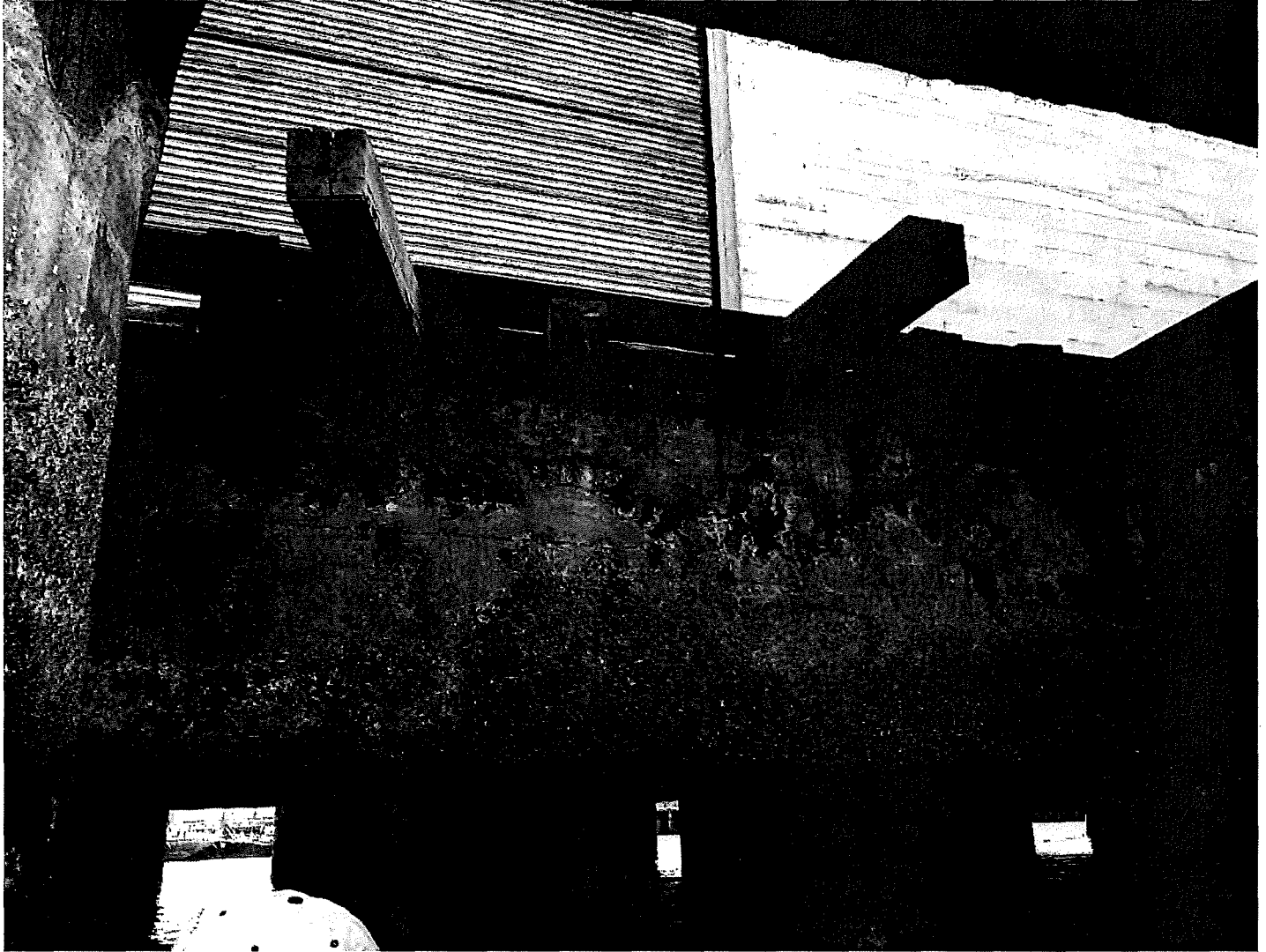
Photo 4. Hole in deck, hanging wood members
