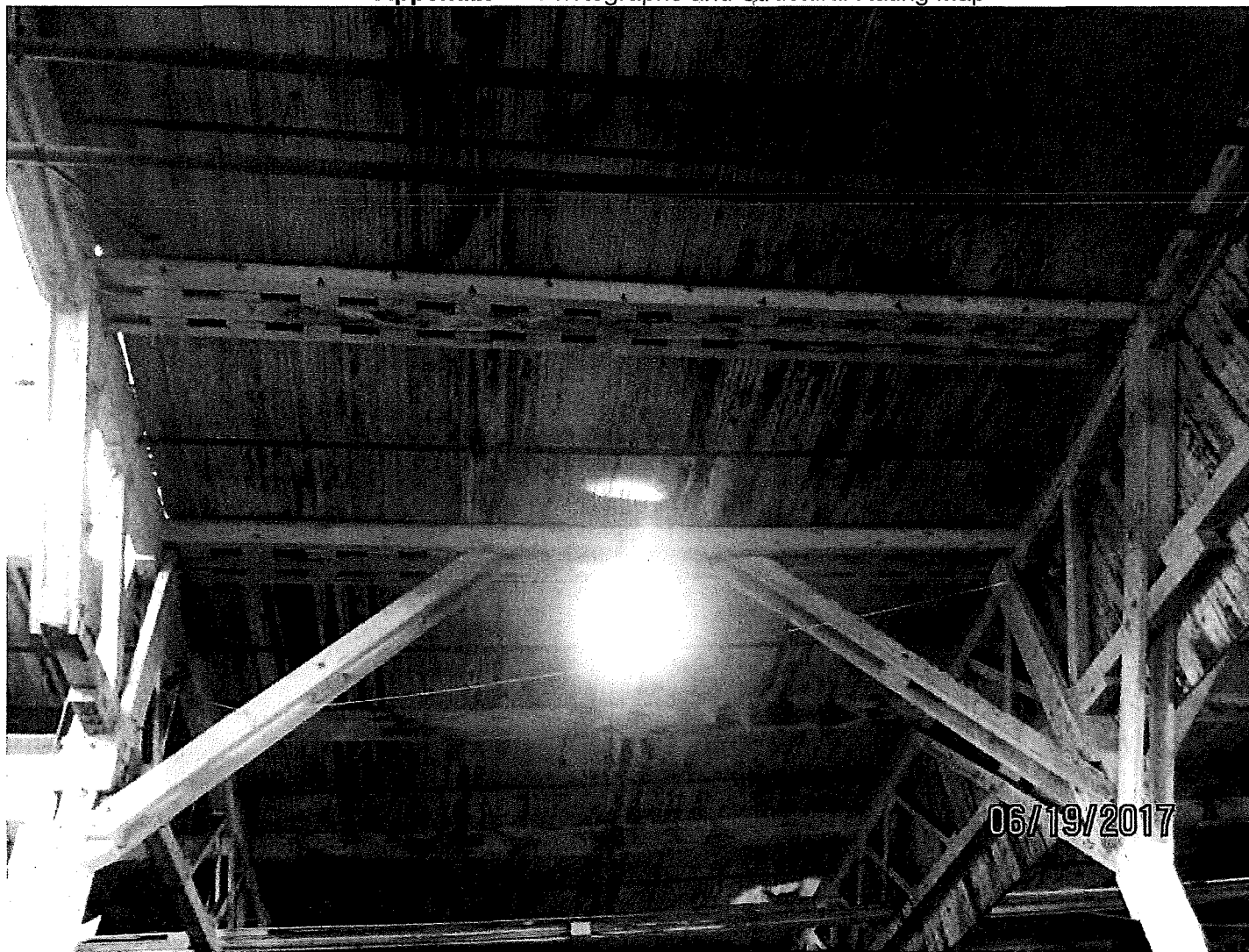
Photo 14. Wood roof beams strengthened in the past.
