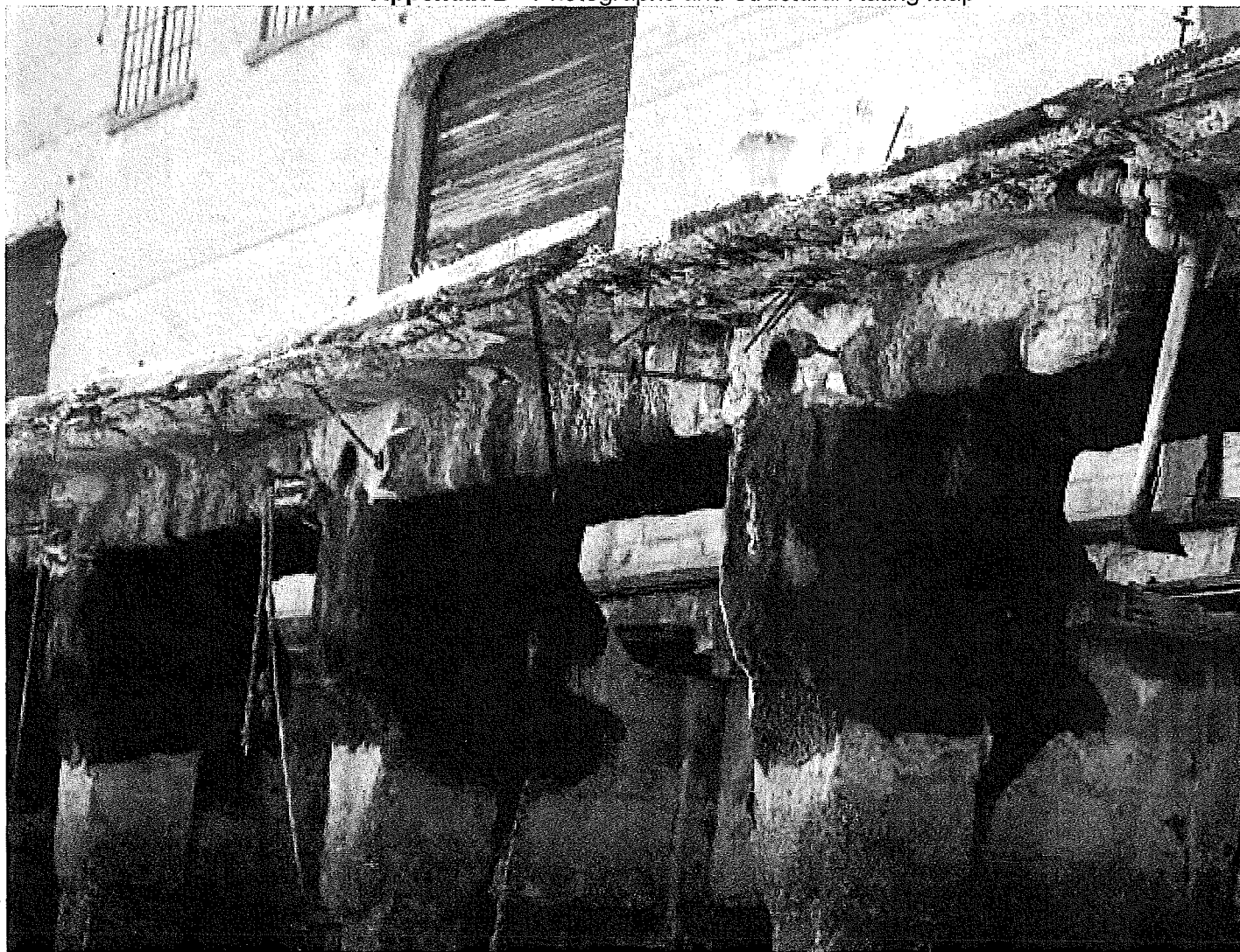
Photo 9. Deteriorated deck
