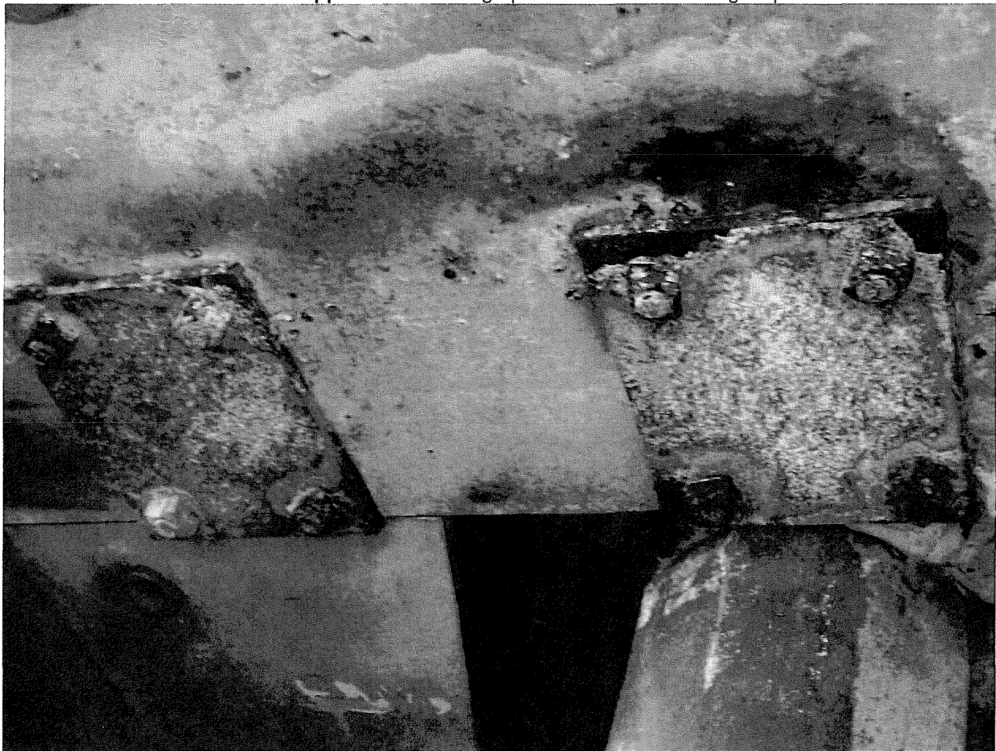
Photo 7. Corrosion on steel plates
