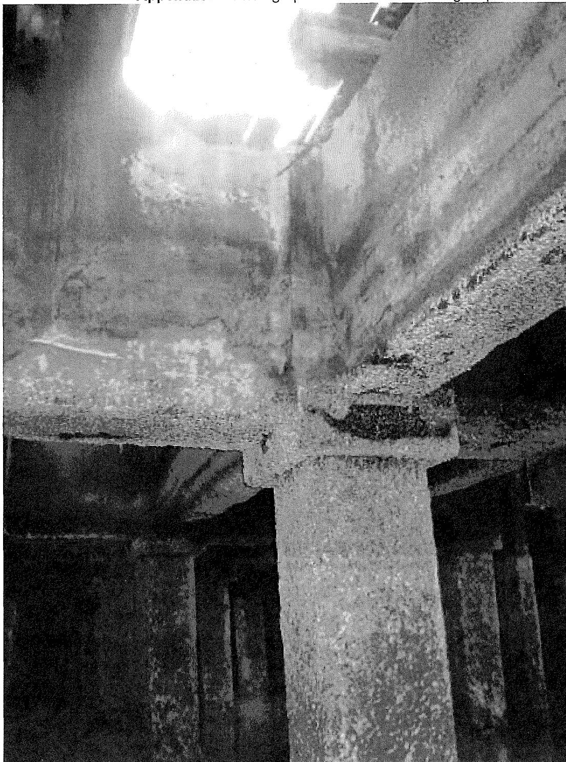
Photo 4. Hole at deck
