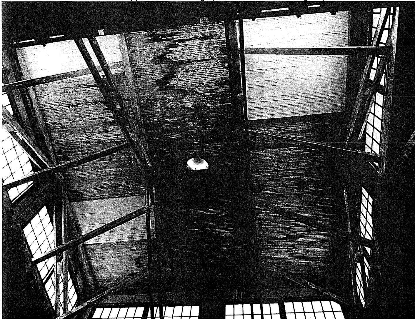
Photo 6. View of a roof pop-up area with shoring work on wood beams. Note water intrusion stains on roof sheathing
