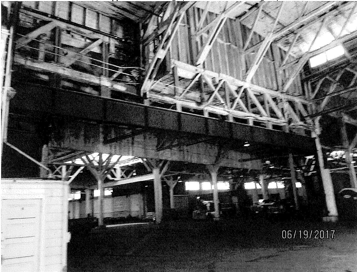
Photo 7. New steel beam and tube steel posts added in 2017 to strengthen existing wood truss.
