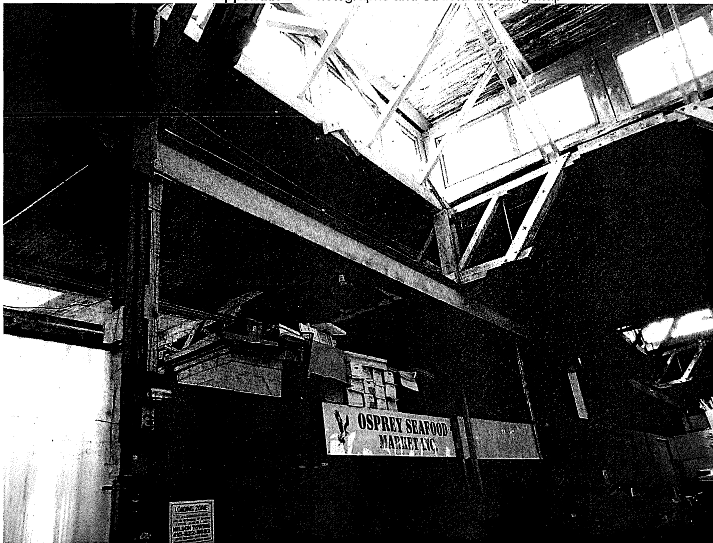
Photo 5. View of roof repair work at the fire damaged area. Note: A steel beam replaces a removed wood post due to fire
