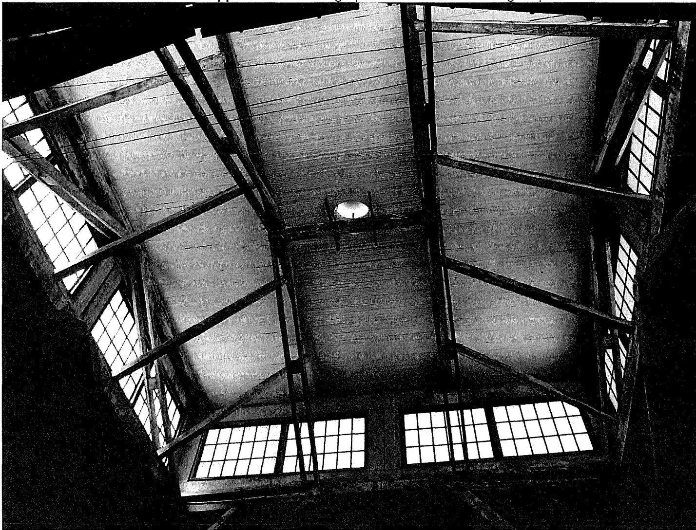
Photo 8. View of a timber roof pop-up area with shoring work on wood beams and replaced roof sheathing
