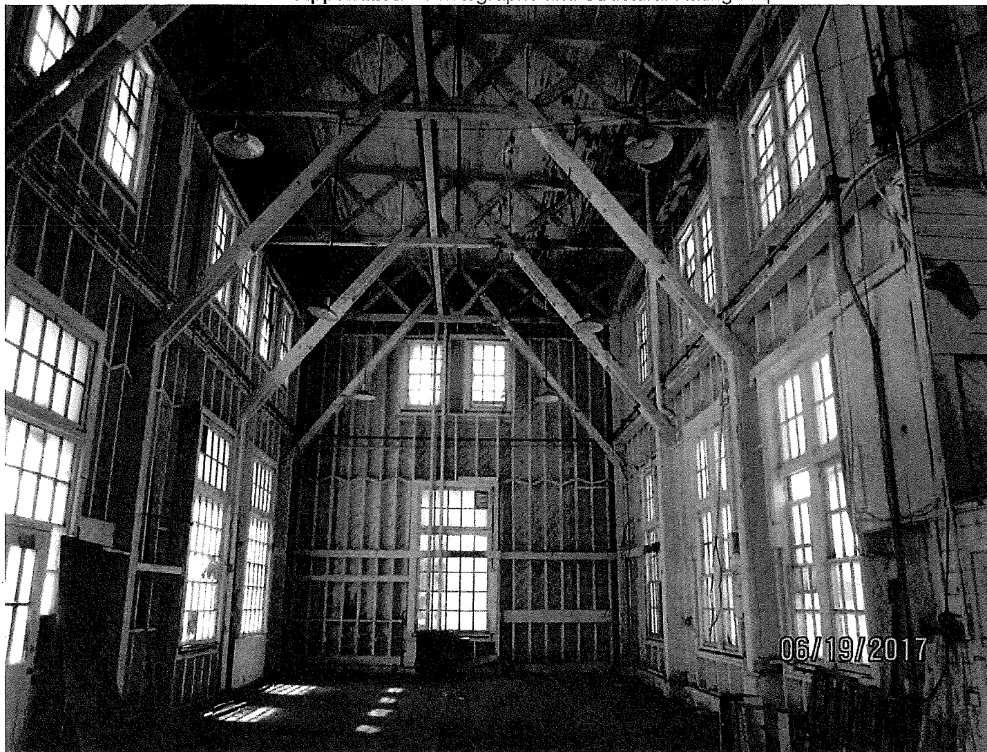
Photo 5. Typical bulkhead framing.
