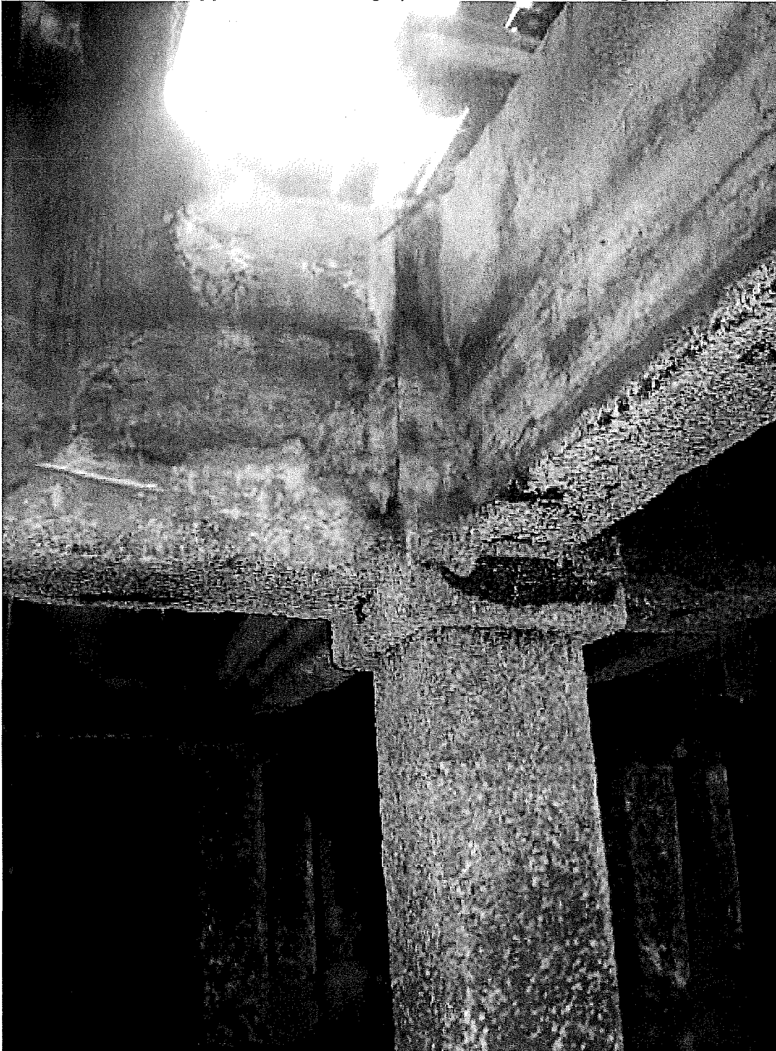
Photo 4. Hole at deck
