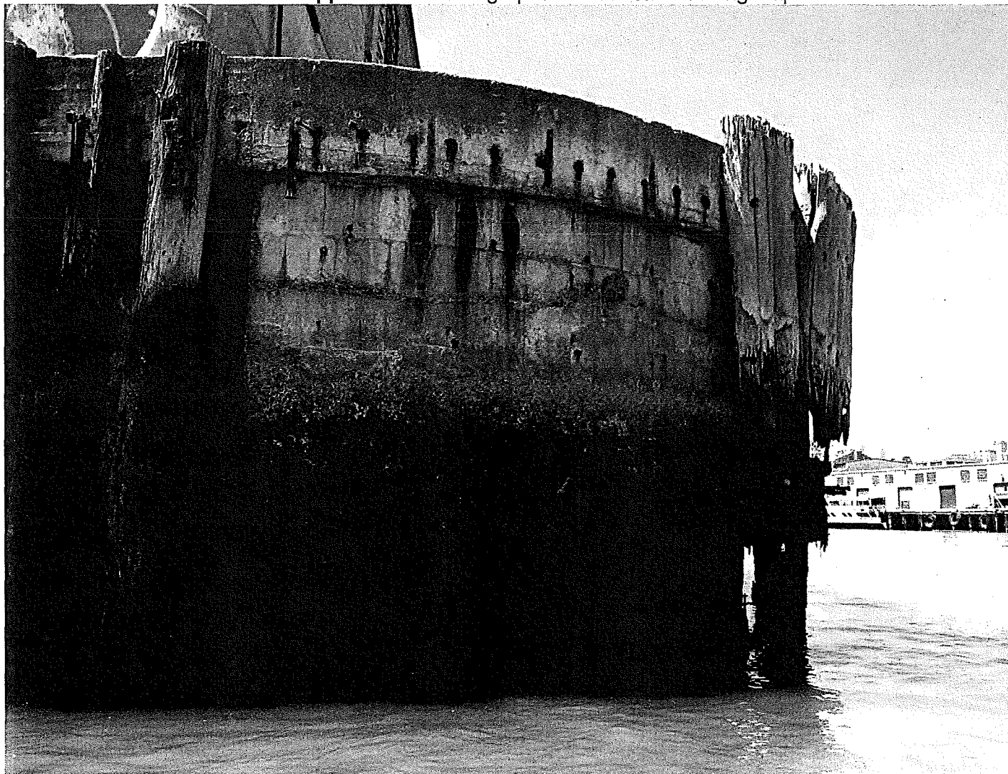
Photo 3. Deteriorated wood piles at pier corner
