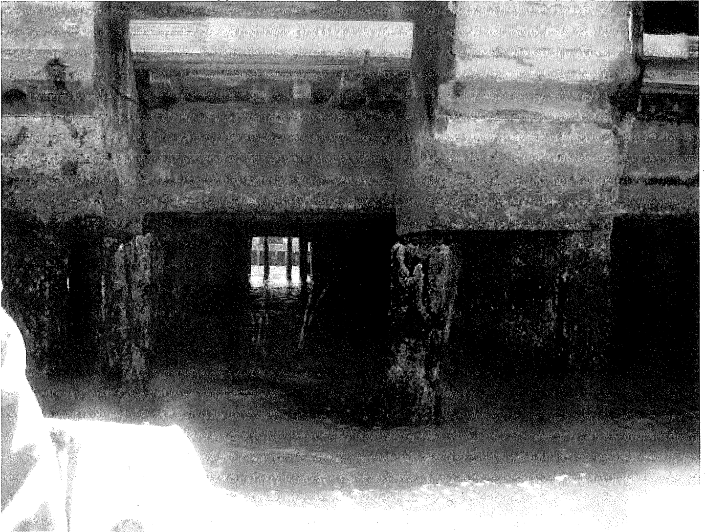
Photo 5. Deteriorated fender piles
