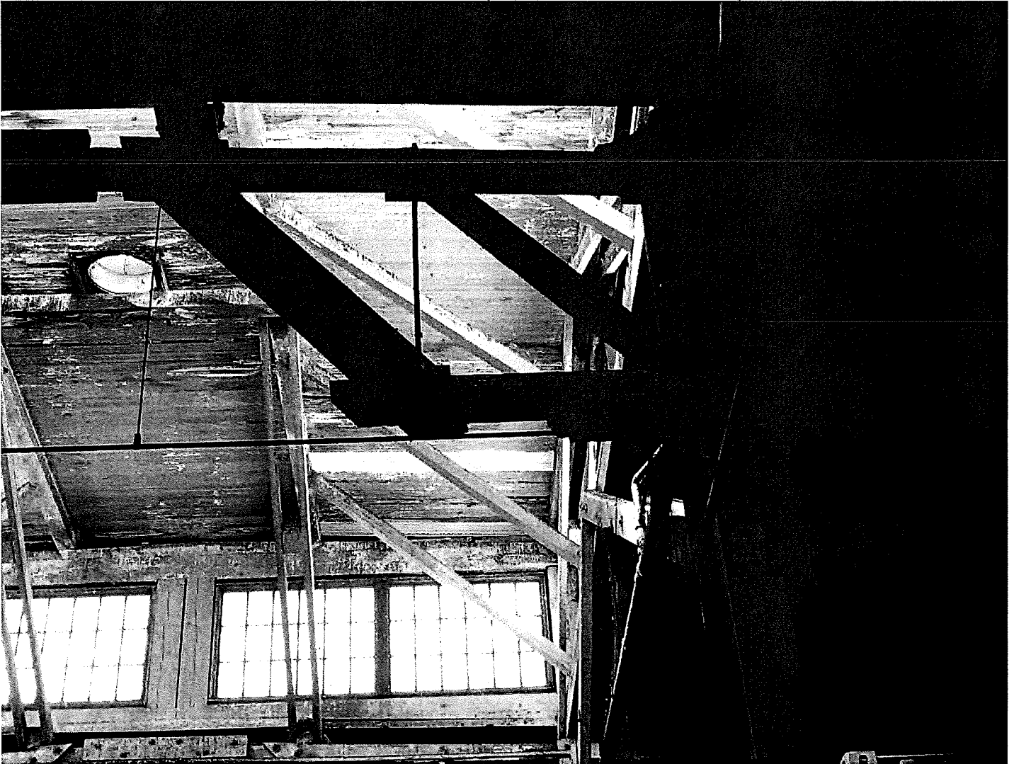
Photo 13. View of a modified timber roof truss. Note the water staining in the roof sheathing beyond
