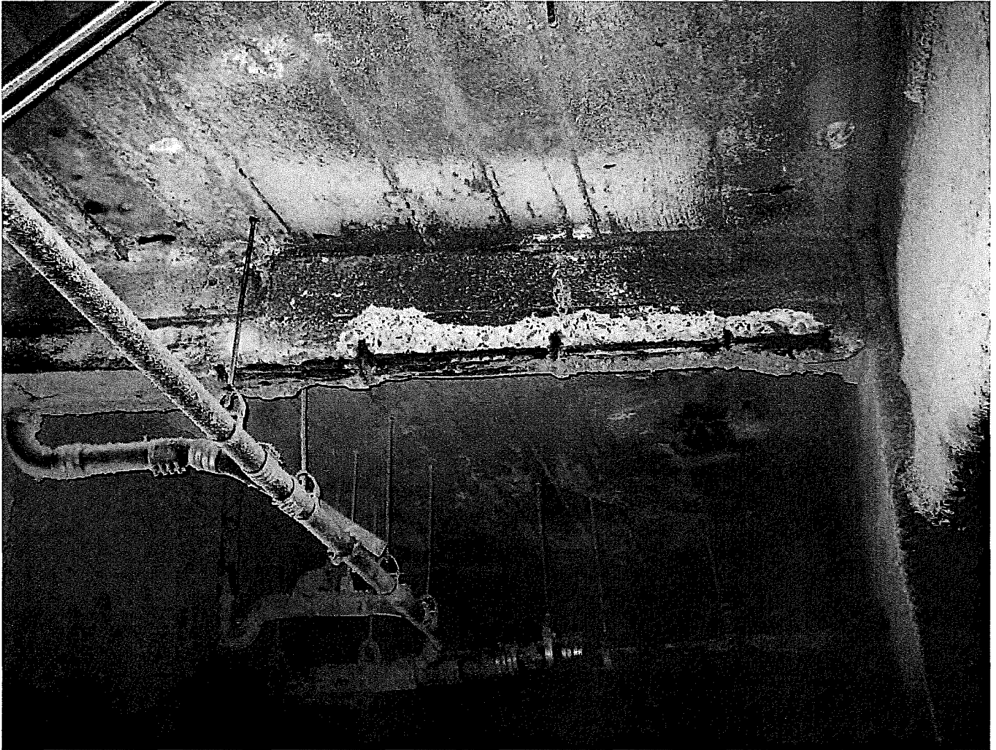
Photo 6. Spalling and exposed/corroded rebar on beam
