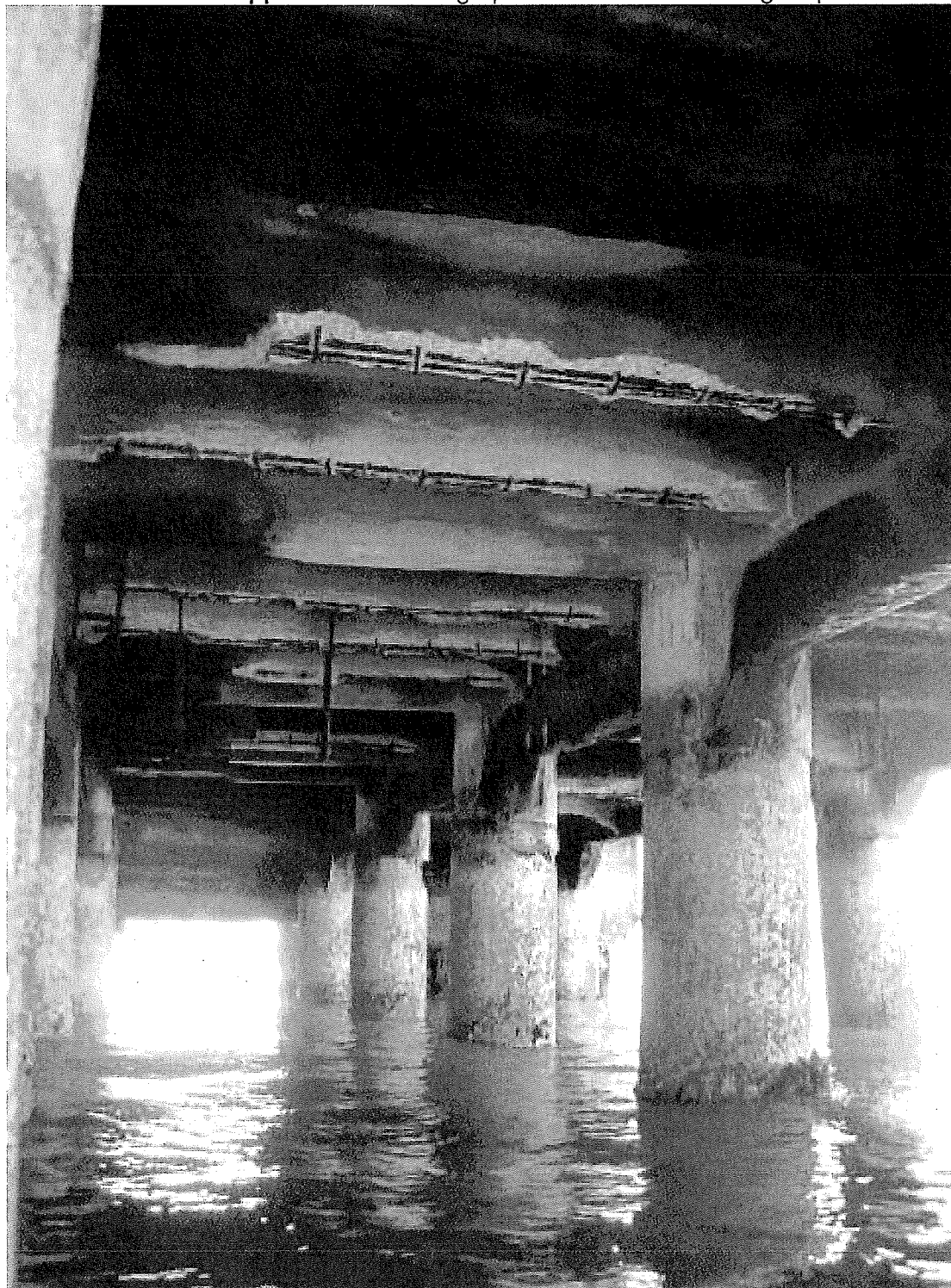
Photo 5. Spalling of concrete beam with exposed/corroded rebar
