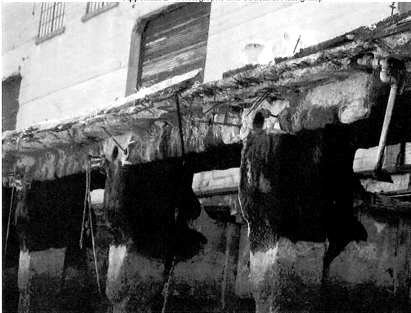
Photo 9. Deteriorated deck
