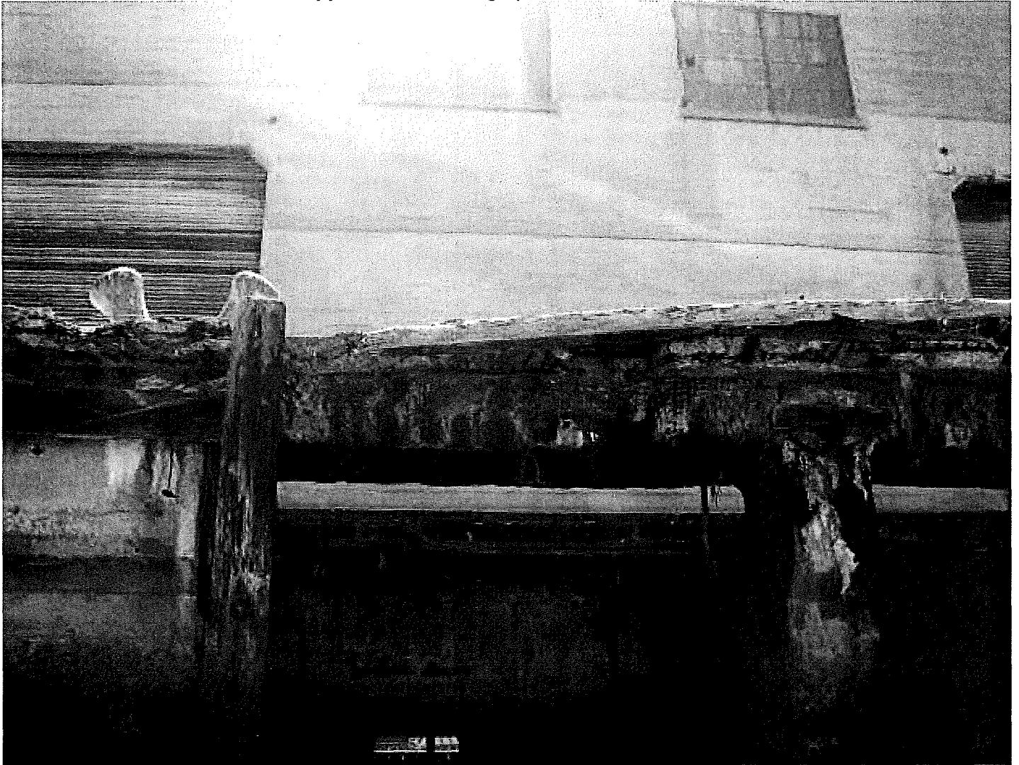
Photo 10. Spalling deck and corroded/exposed rebar
