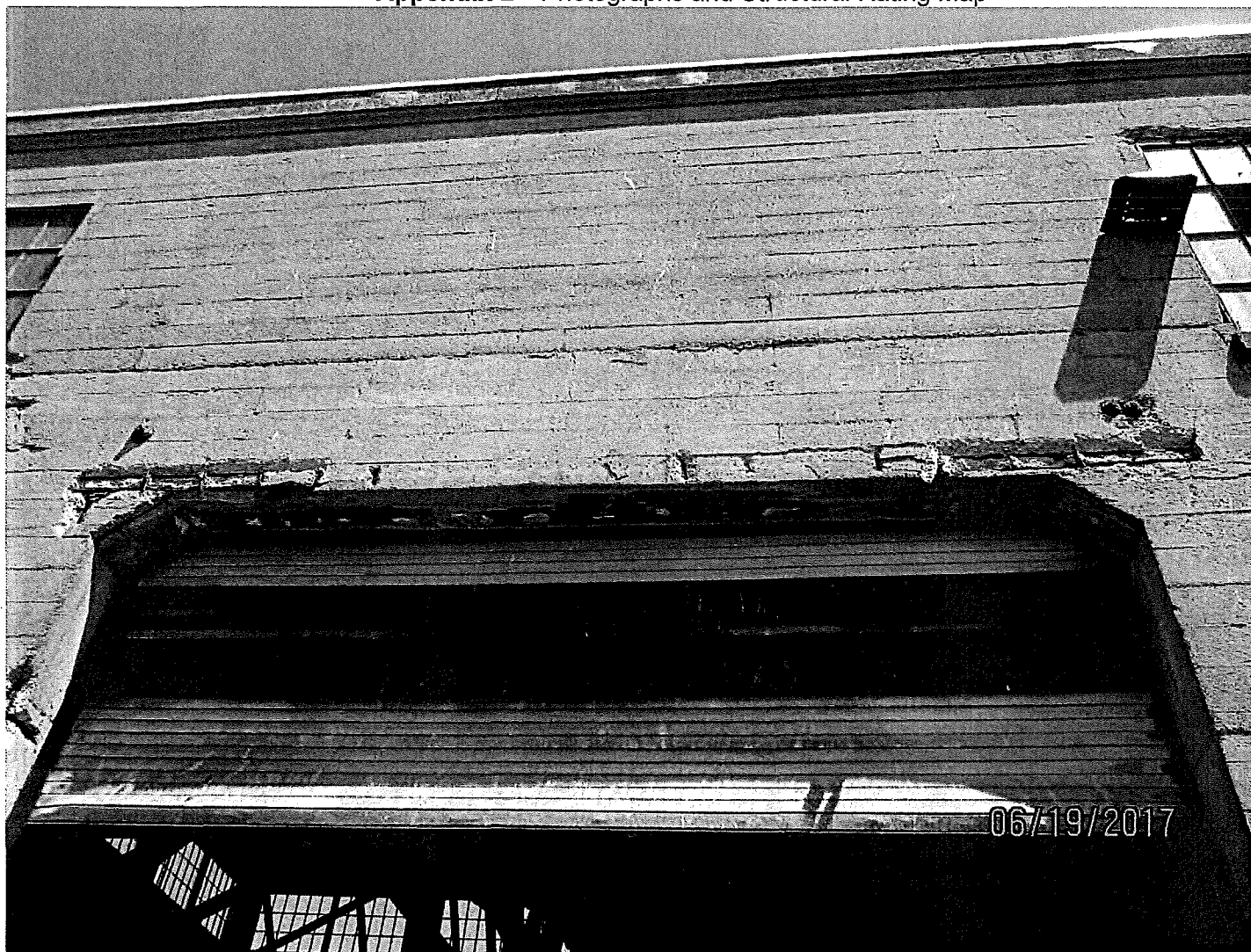
Photo 4. Spalls around roll-up door opening on north face wall. Repairs are planned as part of a future project.
