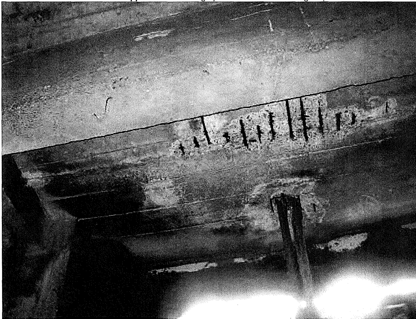
Photo 1. Spalling and corroded/exposed rebar at slab
