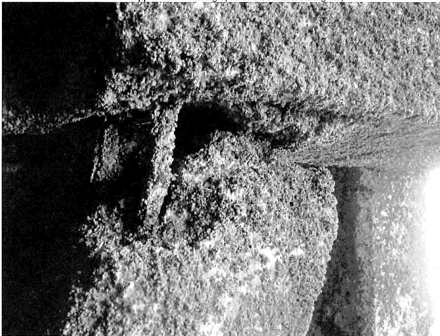
Photo 11. Close up of broken batter pile
