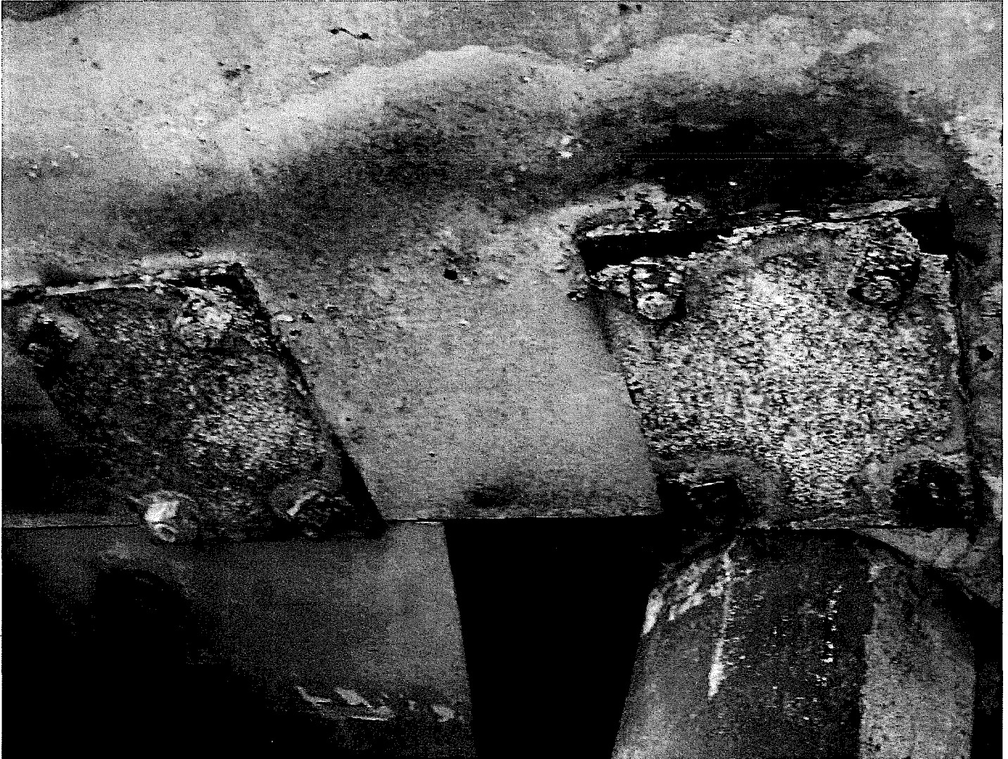
Photo 7. Corrosion on steel plates
