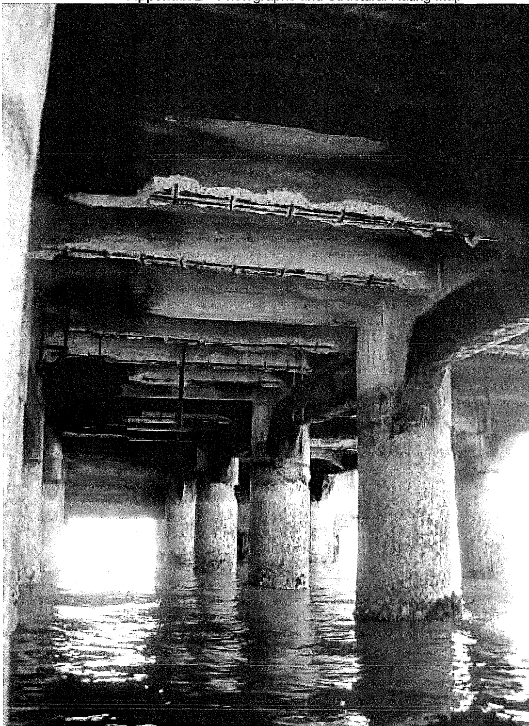
Photo 5. Spalling of concrete beam with exposed/corroded rebar
