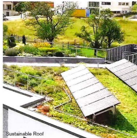
Green Roof Integrated Photovoltaic System
