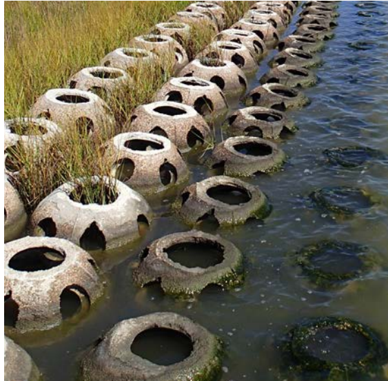
Reef Balls provide shoreline protection and niche habitats
