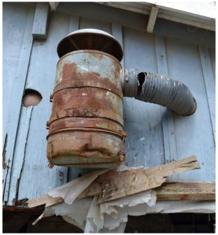
Figure 46. Detail of mounted ventilator
