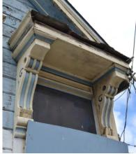
Figure 7. Door hood and bracket detail
