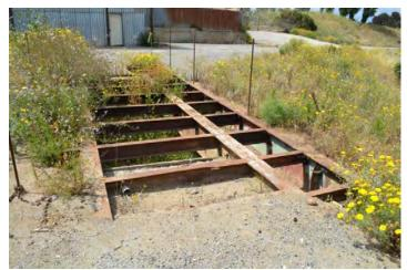
Figure 62. Exposed steel road undergirding, viewed facing northwest
