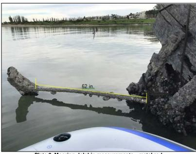
Plate 8. Mooring dolphin measurements—metal rod.
