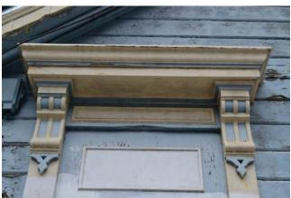
Figure 6. Window transom panel and architrave detail
