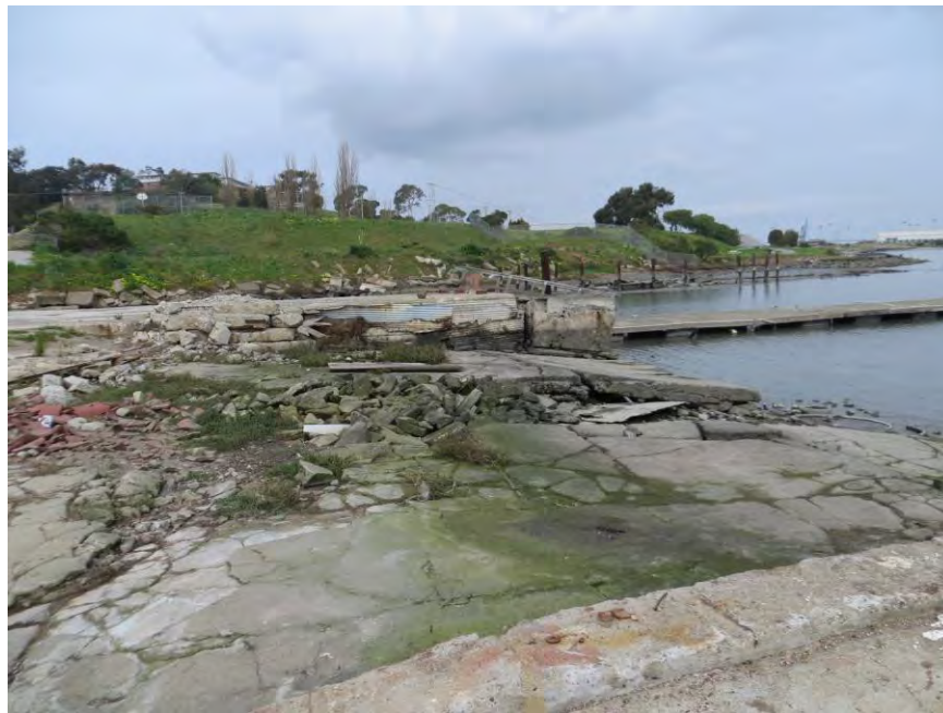
Above: Abandoned house and overgrown shed within the 900 Innes parcel.
