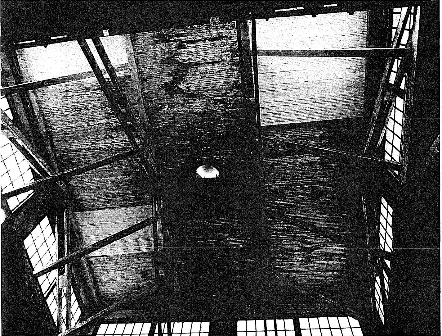
Photo 6. View of a roof pop-up area with shoring work on wood beams. Note water intrusion stains on roof sheathing
