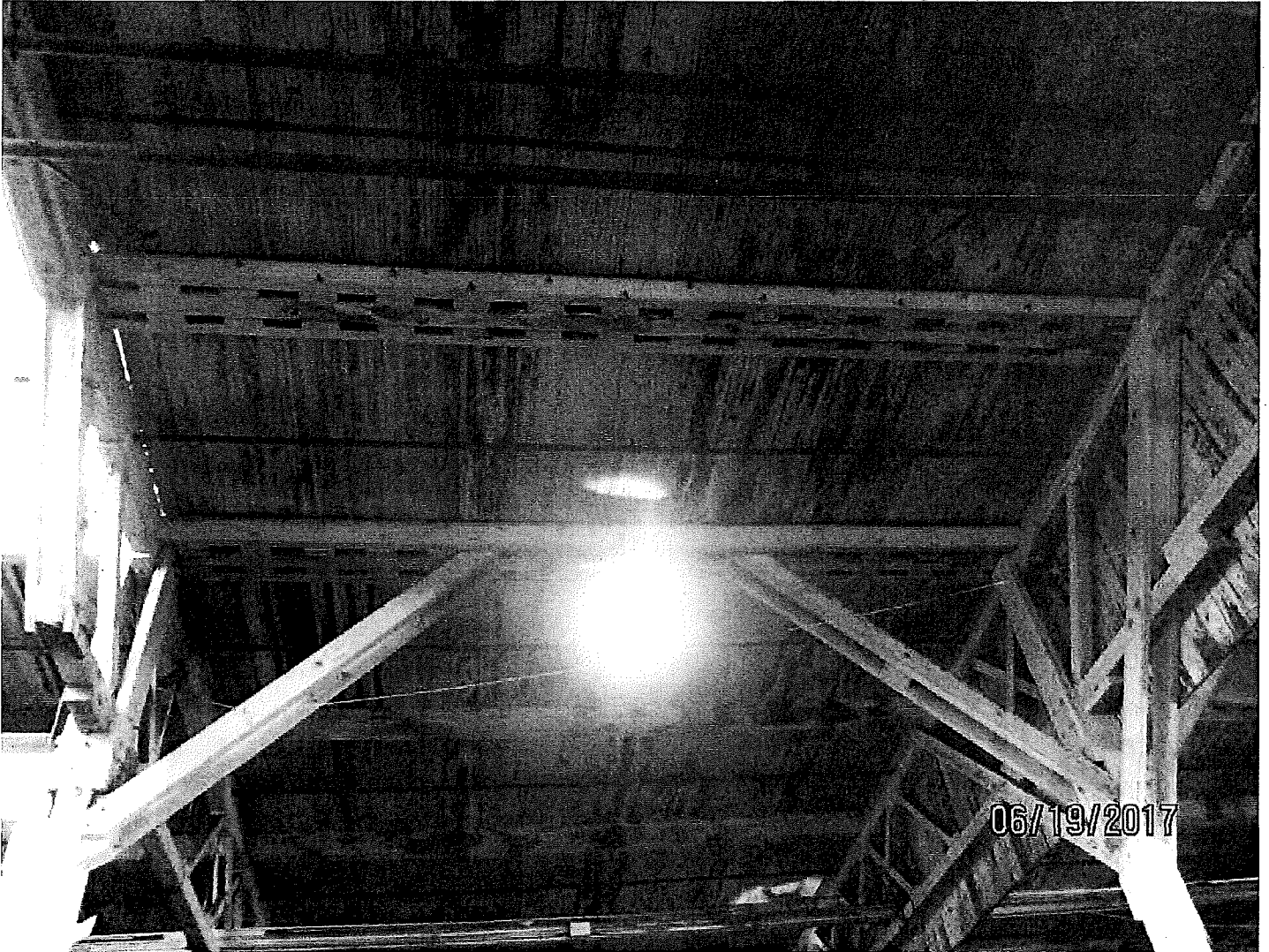
Photo 14. Wood roof beams strengthened in the past.
