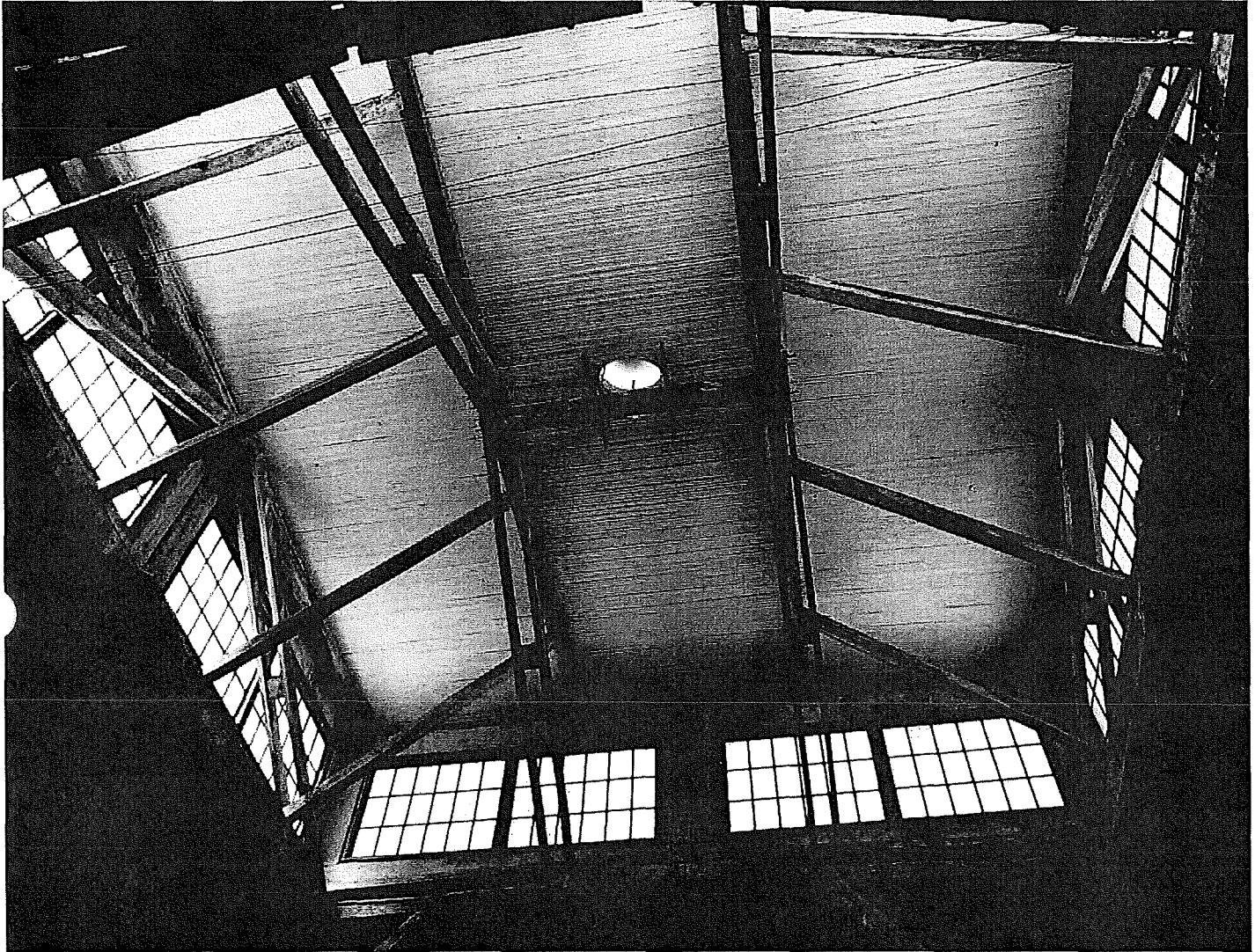
Photo 8. View of a timber roof pop-up area with shoring work on wood beams and replaced roof sheathing
