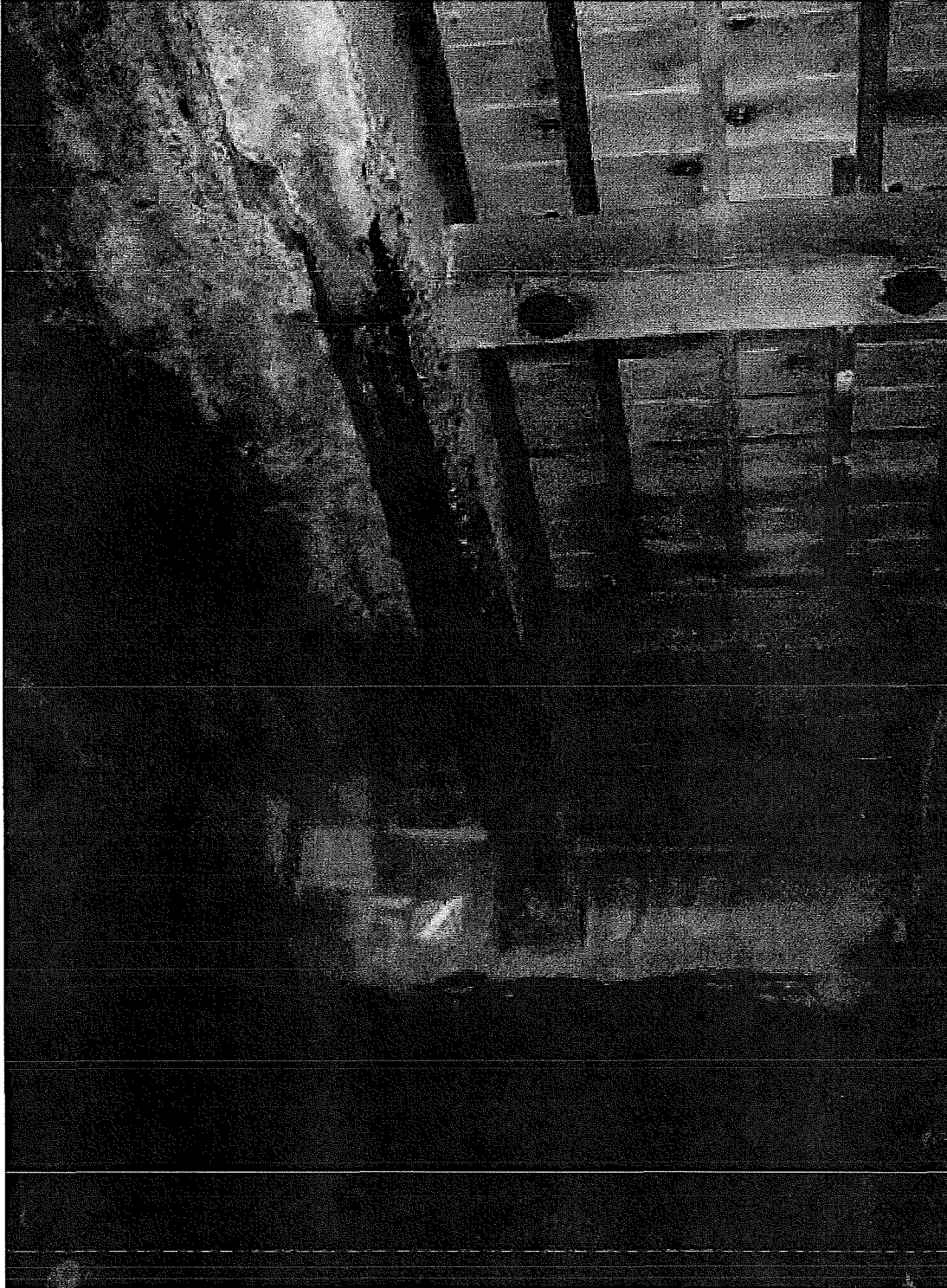
Photo 3. Concrete spalling, typical
