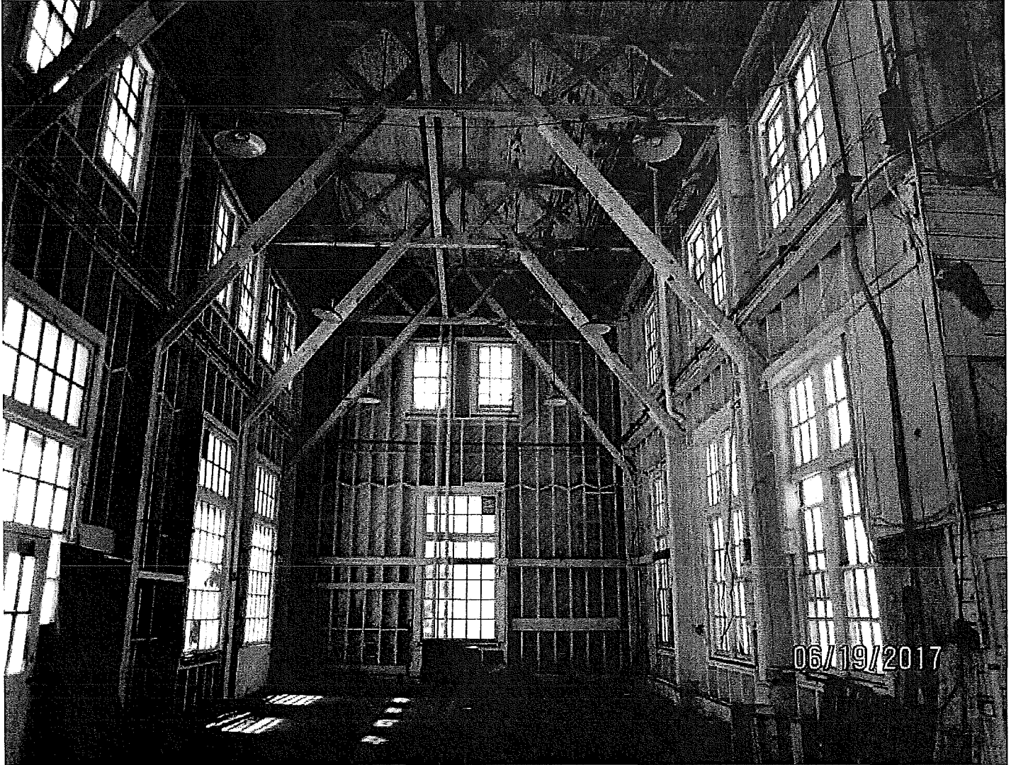
Photo 5. Typical bulkhead framing.
