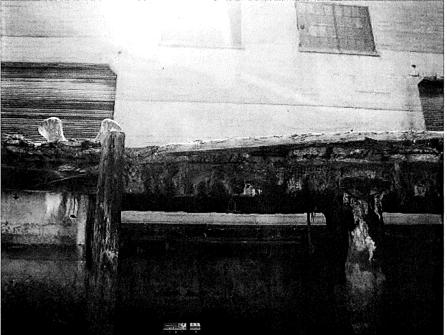
Photo 10. Spalling deck and corroded/exposed rebar
