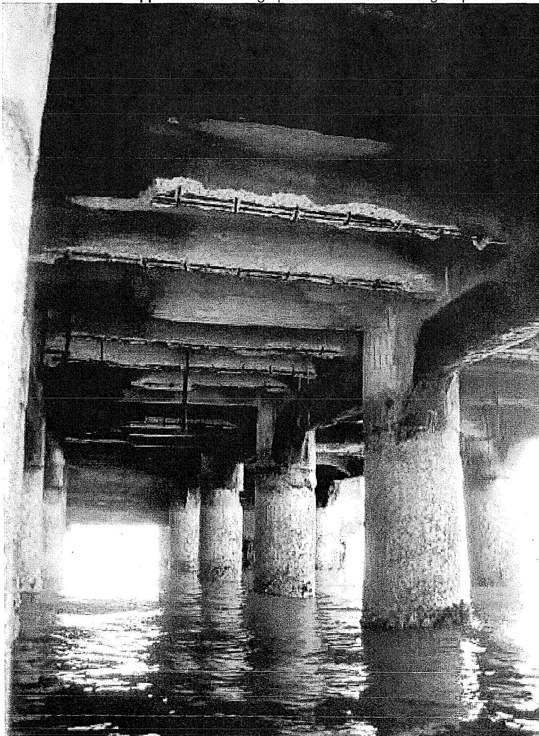
Photo 5. Spalling of concrete beam with exposed/corroded rebar
