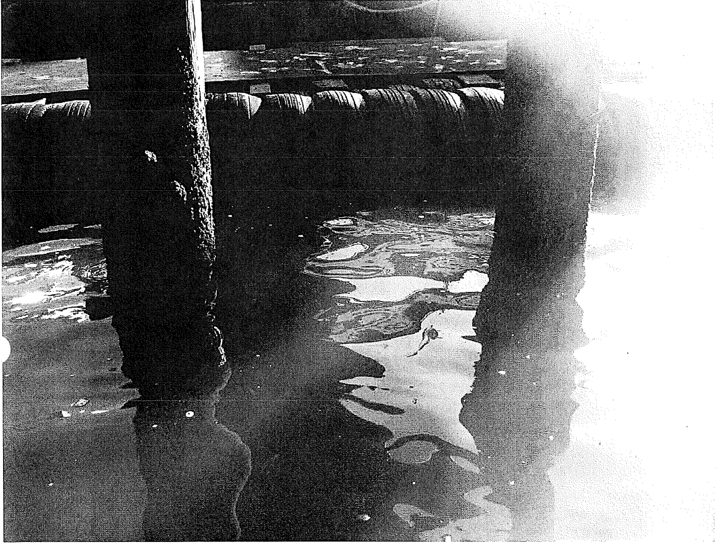
Photo 4. Deteriorated wood piles near metal deck
