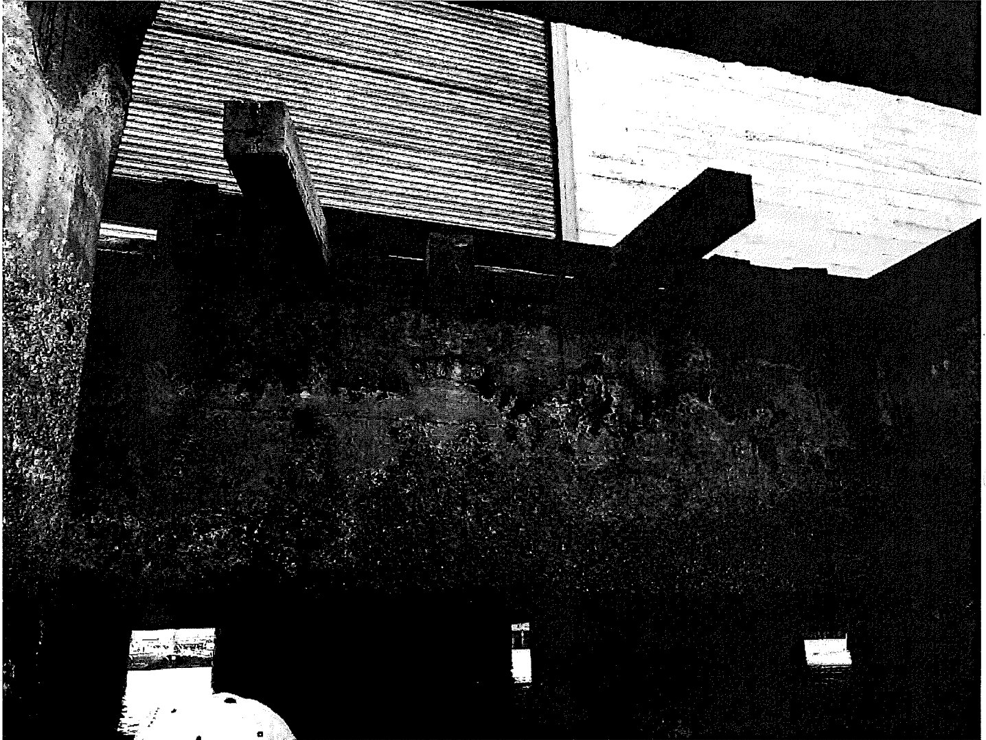
Photo 4. Hole in deck, hanging wood members
