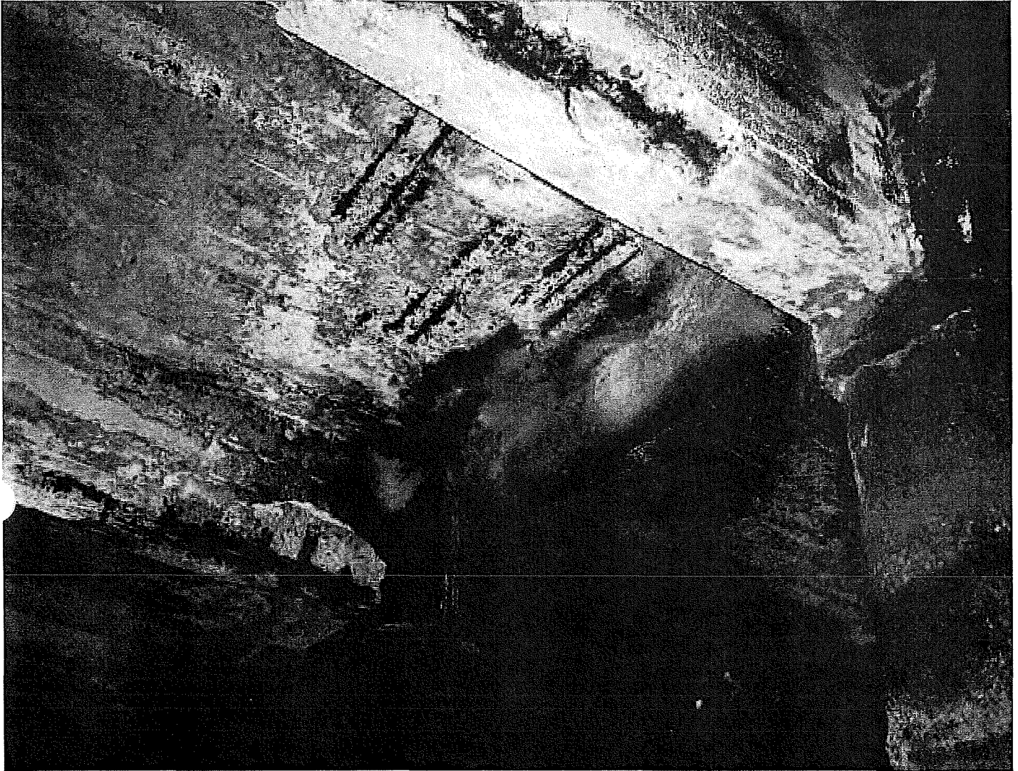
Photo 9. Spalling of concrete beams and slab
