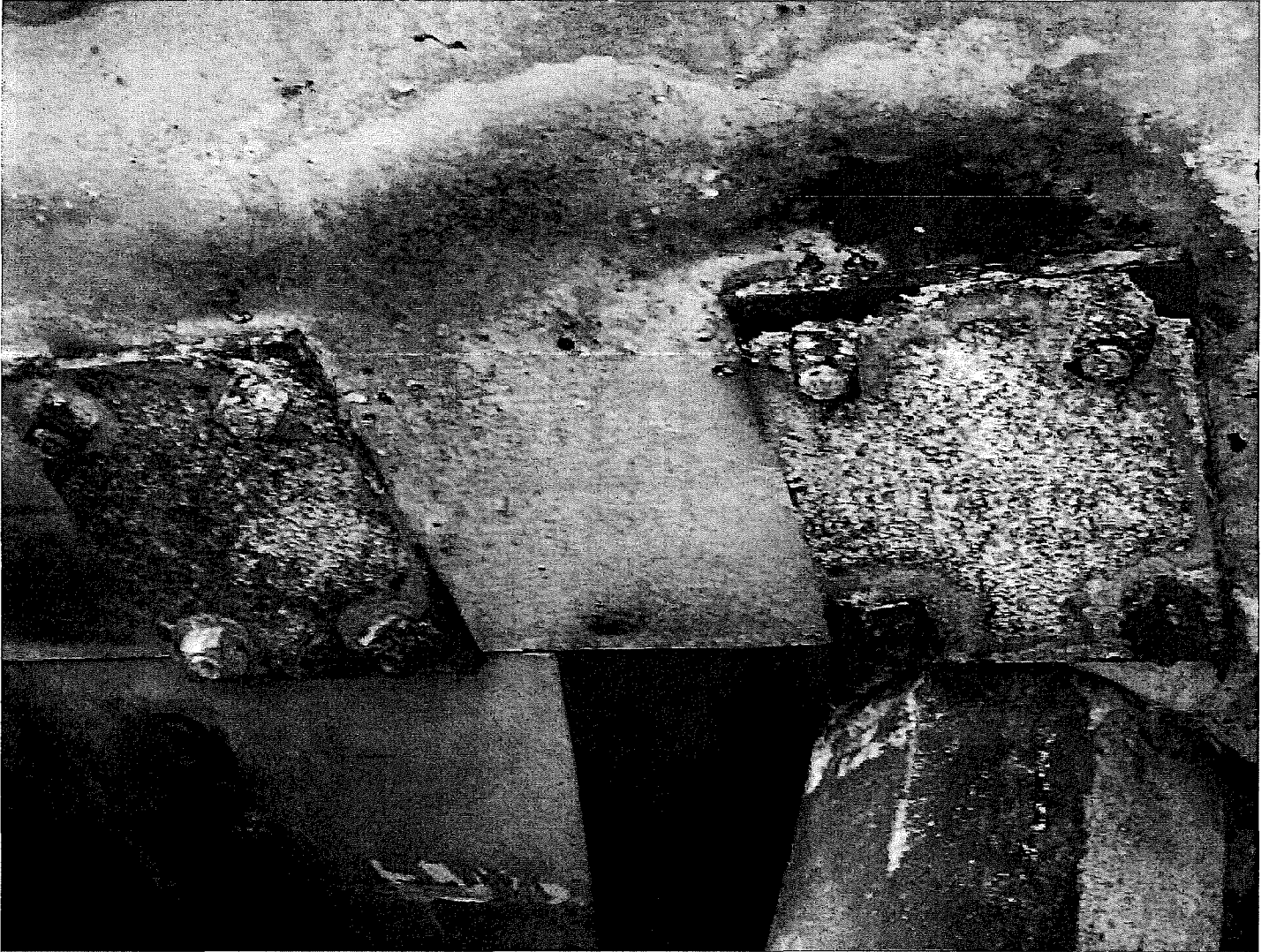
Photo 7. Corrosion on steel plates
