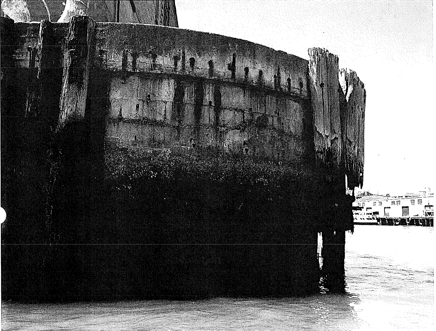
Photo 3. Deteriorated wood piles at pier corner
