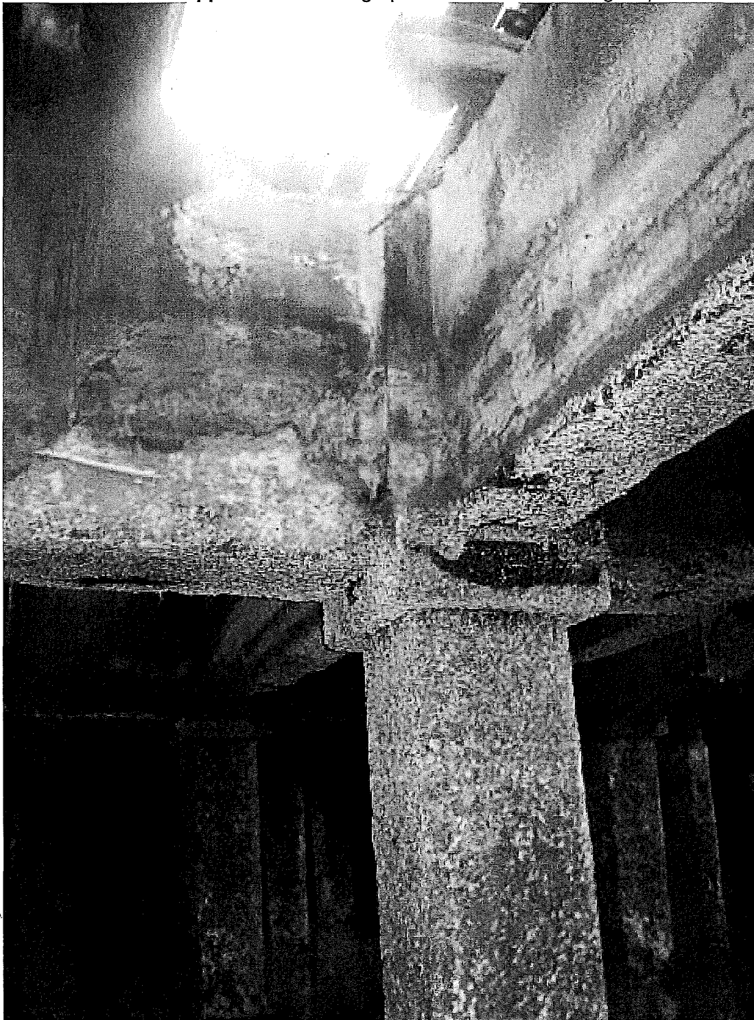
Photo 4. Hole at deck
