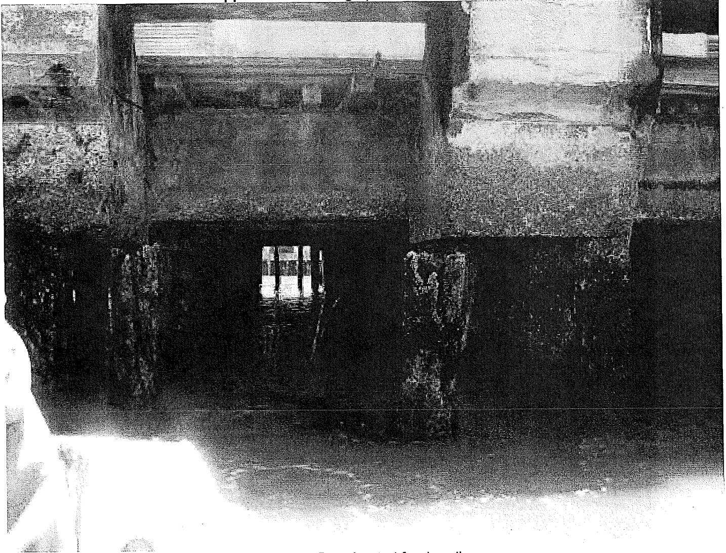
Photo 5. Deteriorated fender piles
