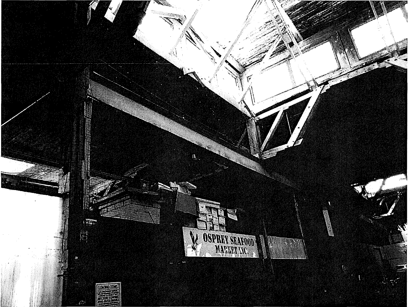
Photo 5. View of roof repair work at the fire damaged area. Note: A steel beam replaces a removed wood post due to fire
