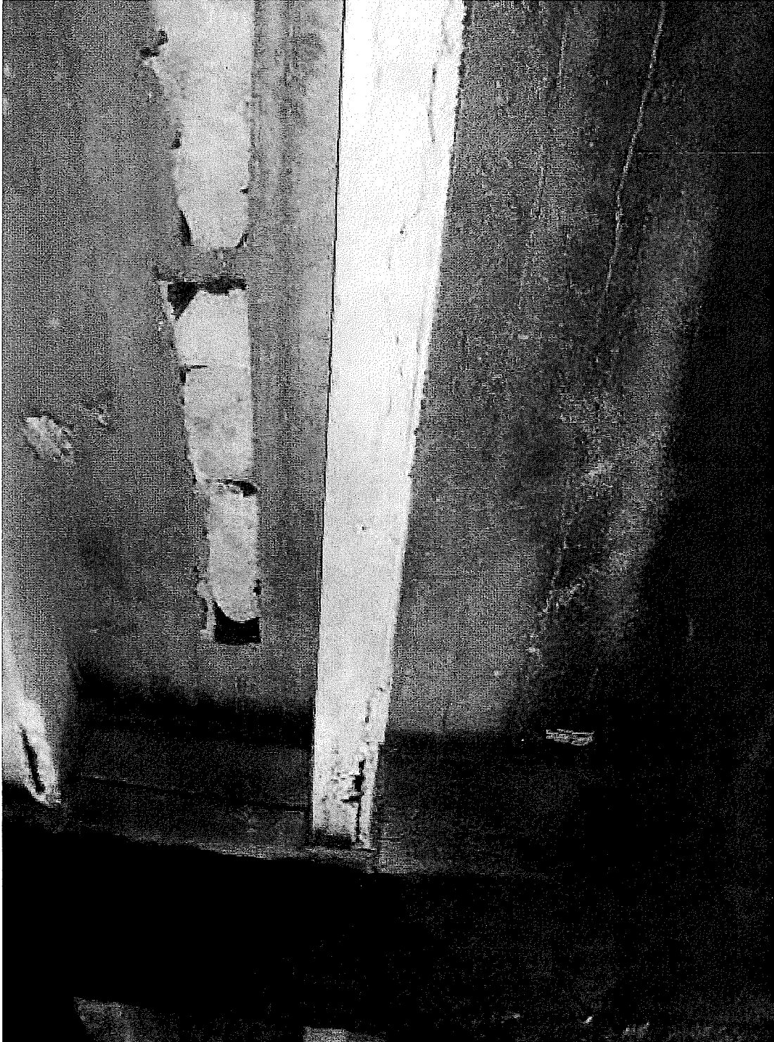
Photo 6. Concrete spalling at slab
