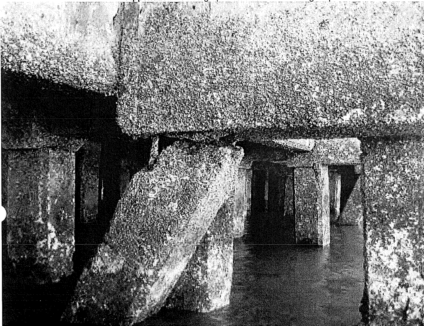
Photo 7. Broken batter pile
