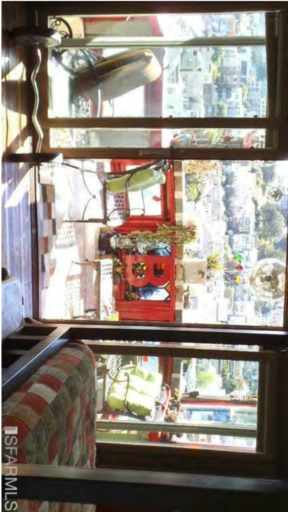
VIEW OF THE TOP FLOOR REAR BALCONY NOTE THE APPROX. 36" HIGH RAILING AND THE DISCO BALLS HANGING FROM THE ILLEGAL REAR ROOF ANWING THAT WAS REMOVED
