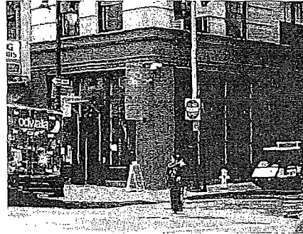
First story storefront. 103_4036.JPG. 3/8/2011
