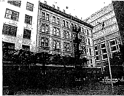
View of southeast facade. 103_4040.JPG 3/7/2011
