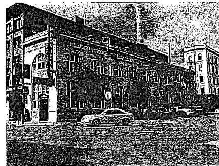
View of southeast and northeast facade. 103_4068.JPG 3/8/2011
