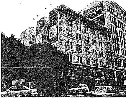
View of northeast and northwest facades. 103_4099.JPG 3/8/2011
