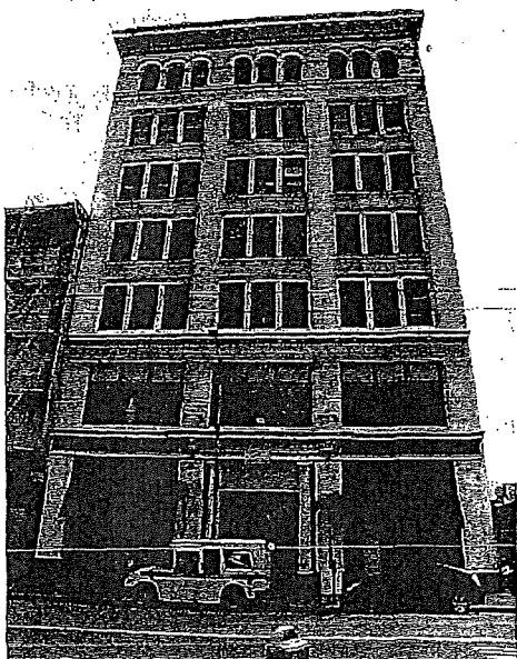
View of northwest facade. 103_4094.JPG; 3/8/2011
