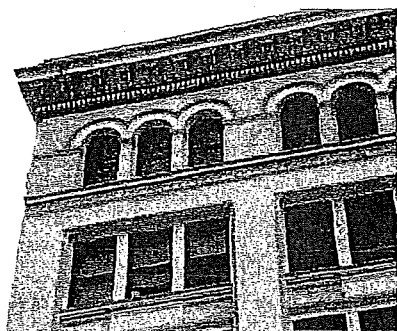
Detail of upper facade. 3/8/2011. 103_4096. JPG
