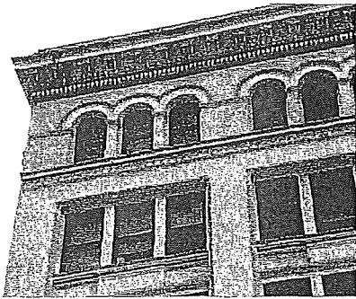
Detail of upper facade. 3/8/2011. 103_4096. JPG
