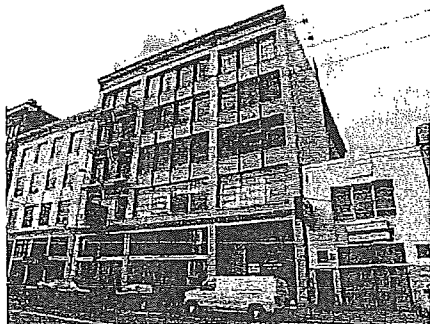
View of southeast facade. 103_4079.JPG 3/8/2011
