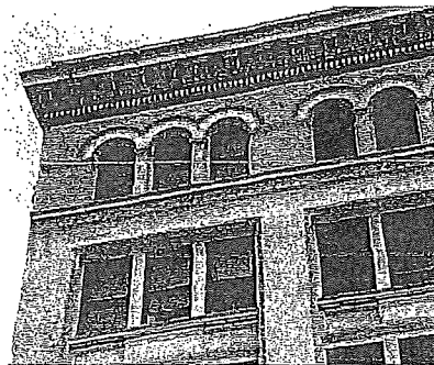
Detail of upper facade. 103_4096.JPG 3/8/2011
