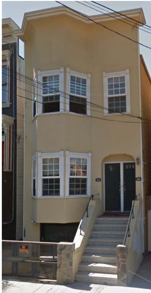
Prior to rehabilitation.
