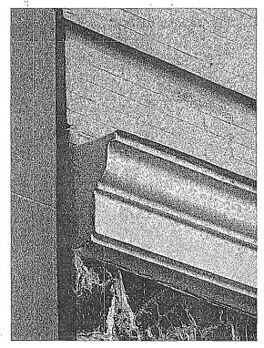
Figure 16: Detail photography of sheet metal water table banding at second floor. Note brick erosion beneath the paint on the brick substrate (photograph taken on 01/26/2018).
