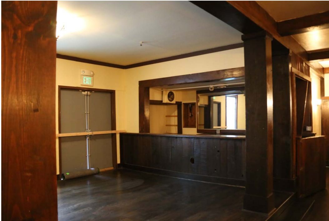
Raised area in rear dining room, view southeast. Note heavy timber framing at left and right.
