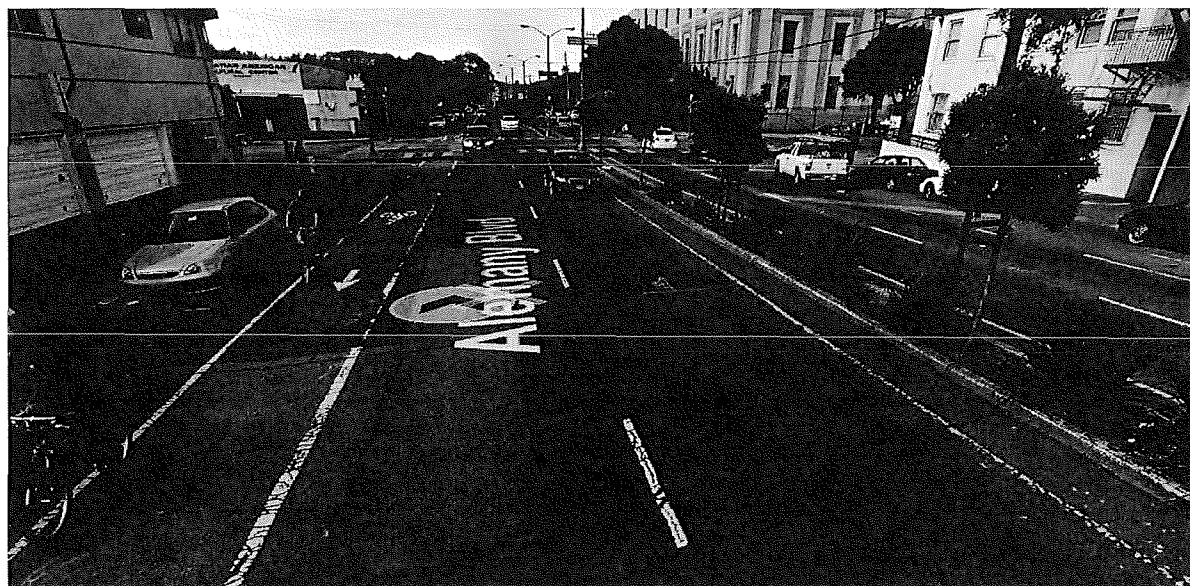
Figure 7: Current Conditions on Alemany Boulevard
