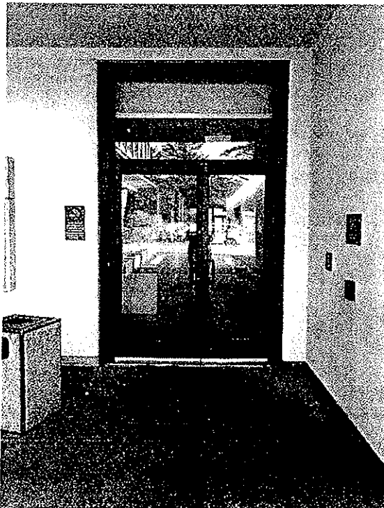
Photo 4: Door from northeast side of the parking lot that leads through the building interior and opens through another secure door into an exterior southeast facing patio area.
