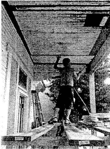
[24] Rotted boards in the beaded-board porch ceiling are being replaced with new matching beaded board.
