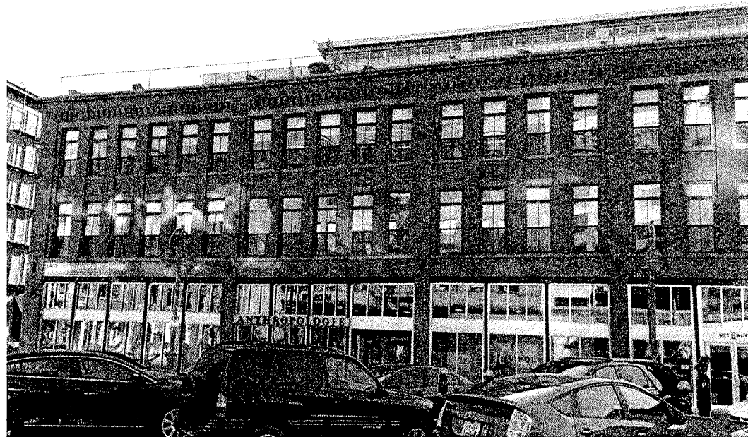
[64] Not Recommended: It is generally not appropriate to construct a rooftop addition on a low-rise, two- to three-story building such as this, because it negatively affects its historic character.
