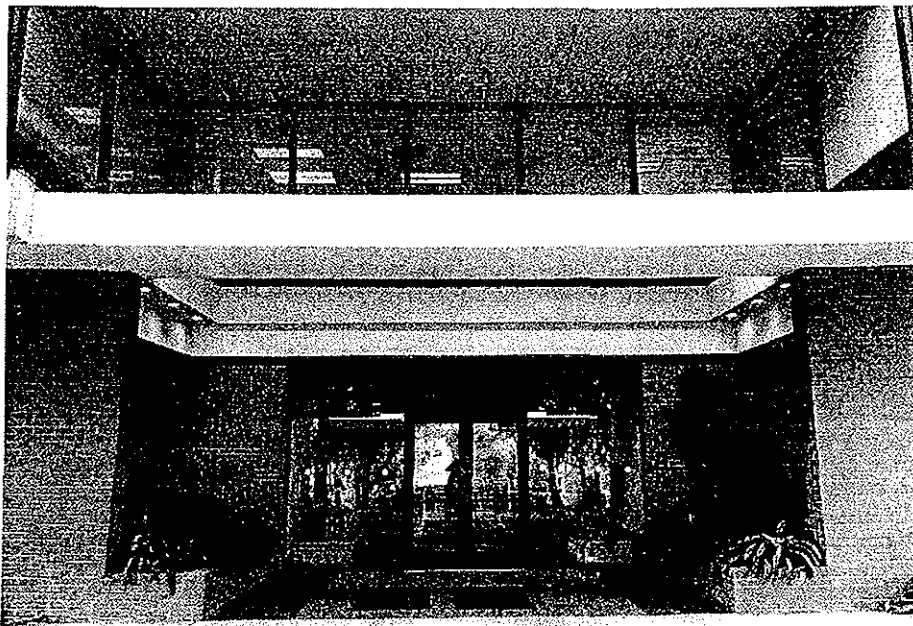
Photo 2: Main Entrance at 3333 California where visitors are required to sign in with the security guard
