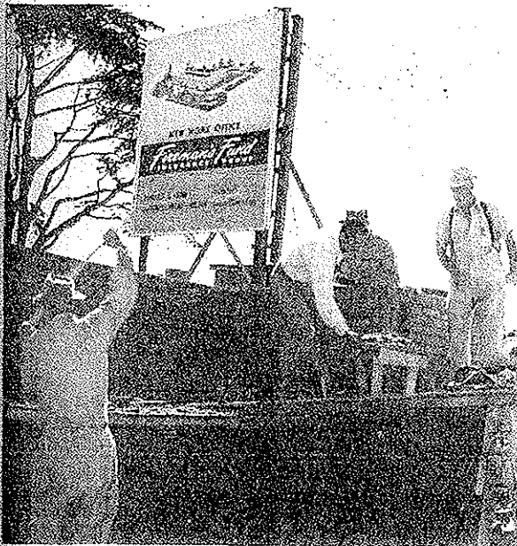
BRICK MASONS doing their part in constructing this modern building.
