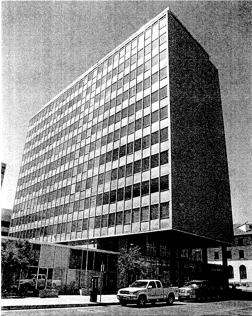
[30] Rather than replace the original curtain wall system of the 1954 Simms Building in Albuquerque, NM, with a different color tinted glass or coat it with a non-historic reflective film, the HVAC system was updated to improve energy efficiency. Photo: Harvey M. Kaplan.
