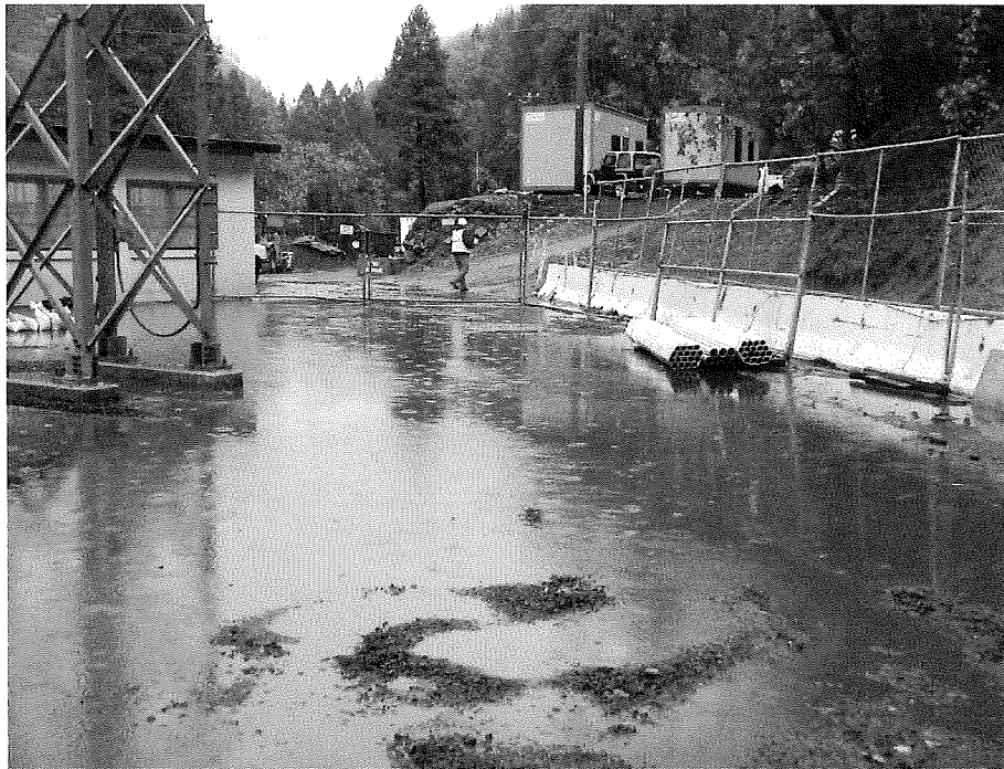
Figure 6. Flooding inside Switchyard near control building (2/28/2014).
