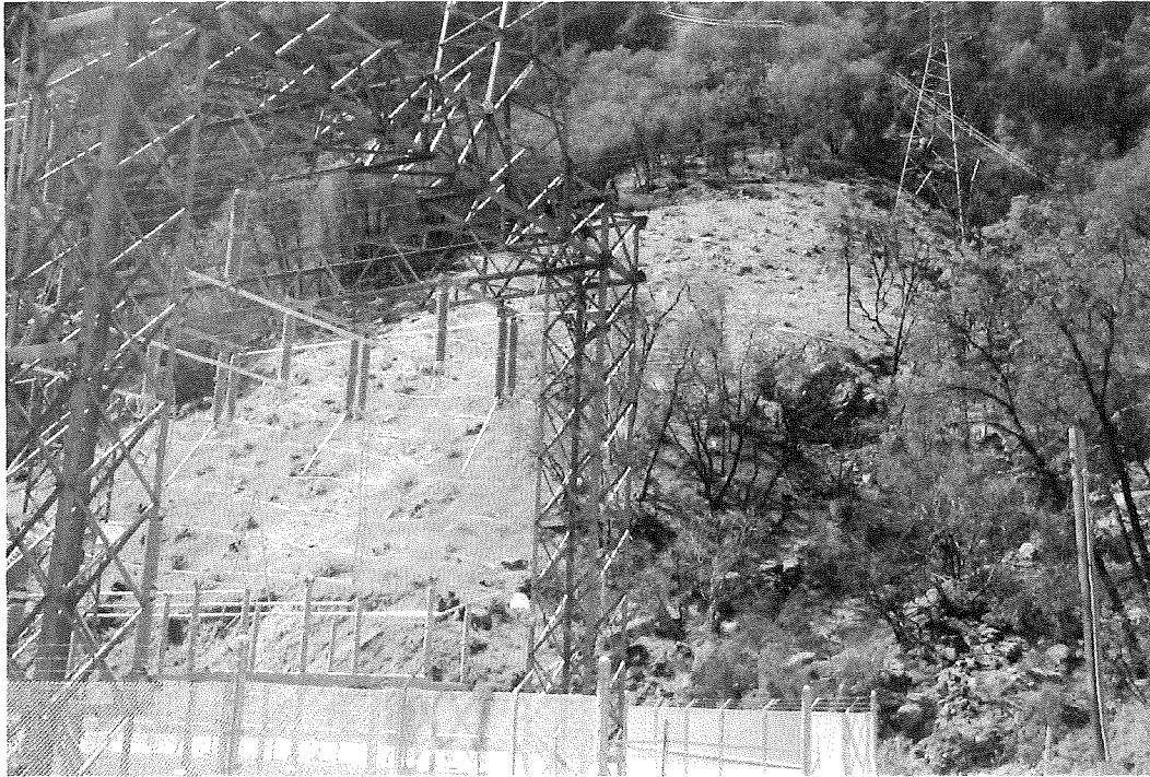
Figure 2-6: Work Area 2 - Steep Slope to the South of ISY Exhibiting Active Raveling Conditions (May 2, 2014)
