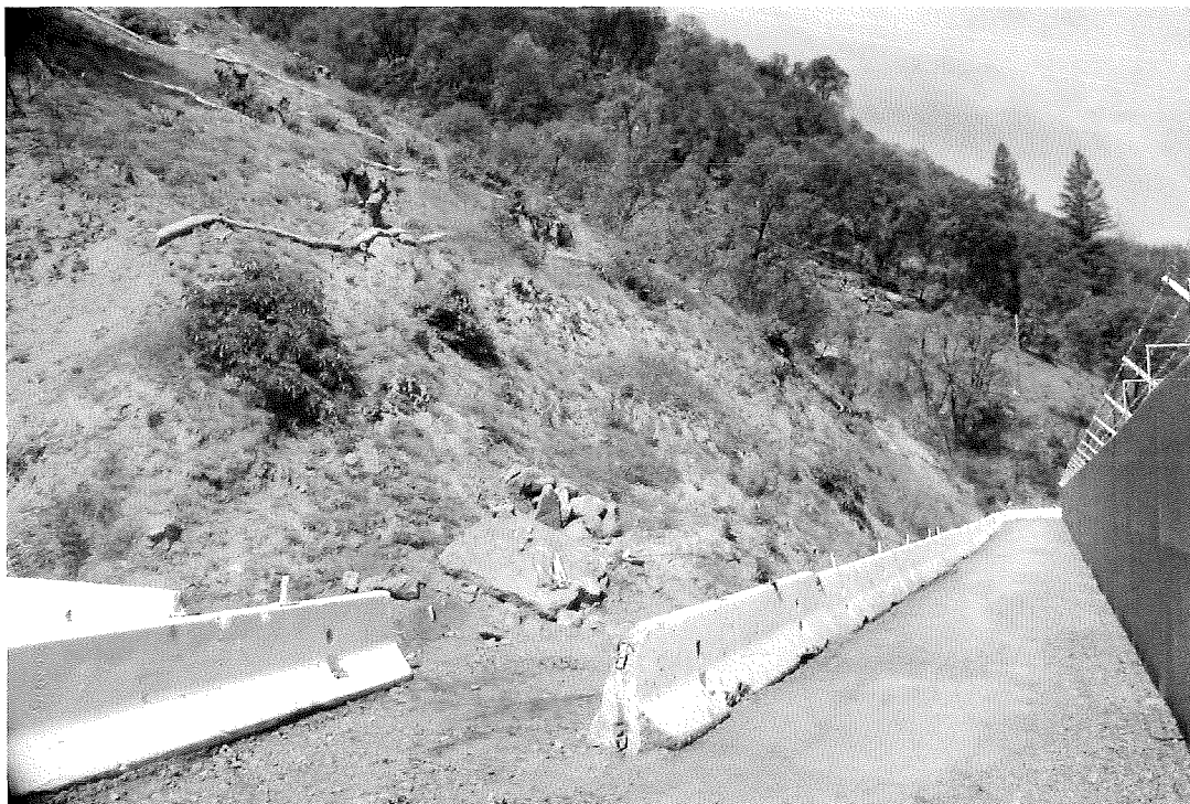
Figure 2-7: Slope Debris from Raveling Slope alongside Access Road on South Edge of ISY (May 2, 2014)
