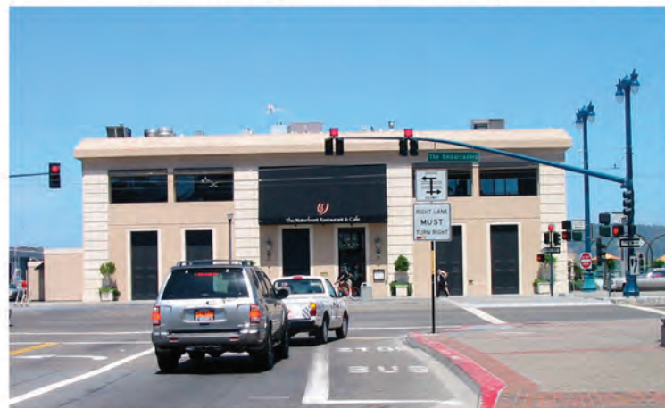
The Waterfront Restaurant & Cafe - Pier 7 & The Embarcadero
