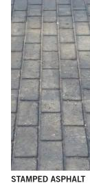
STAMPED ASPHALT VEHICULAR PAVING
