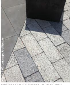
PERMEABLE CONCRETE UNIT PAVERS
