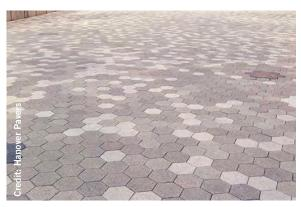
Pre-cast concrete unit pavers and pre-cast permeable concrete unit pavers.
