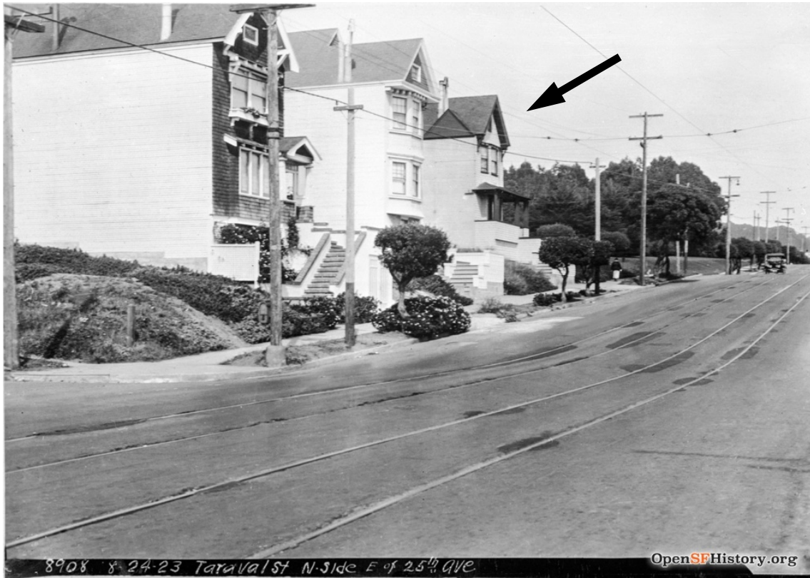
Figure 12: Taraval St looking east circa 1923. Subject property noted with arrow.
