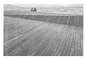
Wood decking made of durable hardwood appropriate for coastal conditions.
