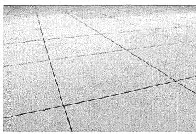
Enhanced cast-in-place concrete with saw-cut joints.
