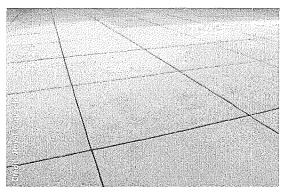
Enhanced cast-in-place concrete with saw-cut joints.
