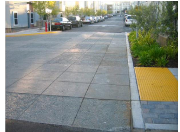
Figure 5.6-5: Raised Street Crosswalk
