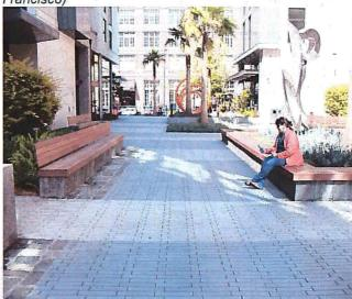
Any porous load-bearing surface that temporarily stores rainwater prior to infiltration or drainage to a controlled outlet.
