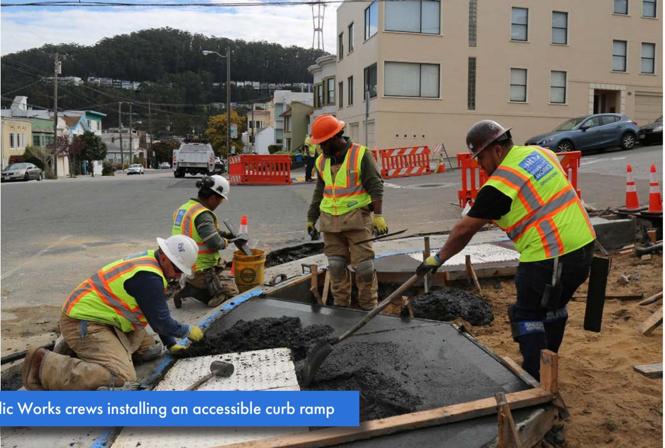
Public Works crews installing an accessible curb ramp
