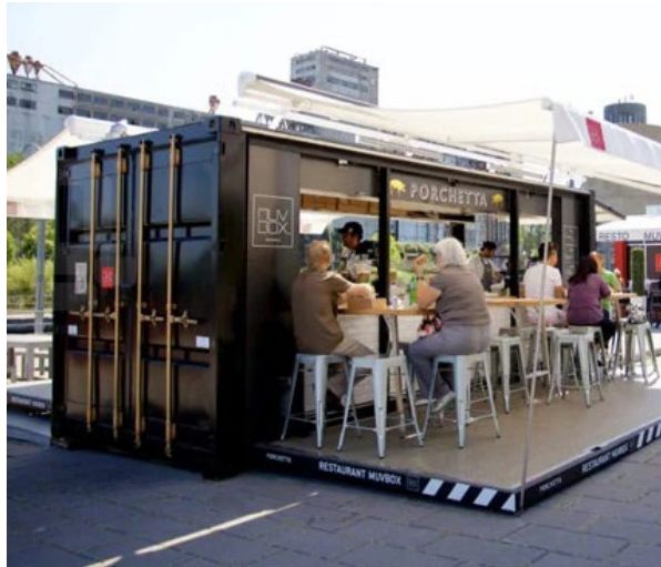
Prefabricated shipping container kiosk
