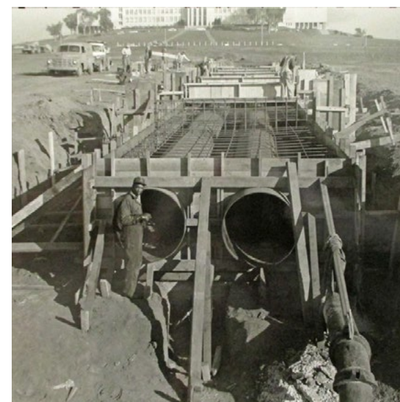
Balboa Reservoir Inlet/Outlet Pipes, 1957
