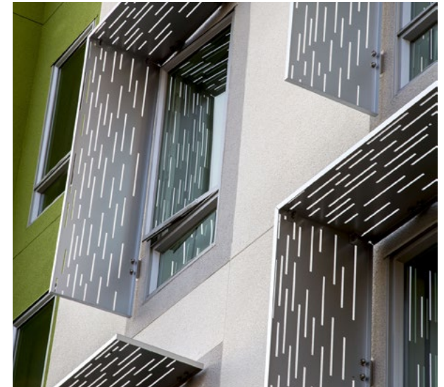
Sunscreens to reduce solar gain
