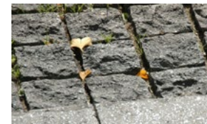
Cobble stone with split sides and flamed top or split top and sides
