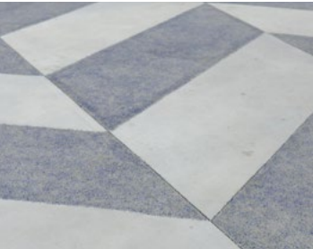
P2: cast-in-place concrete with seeded aggregate
