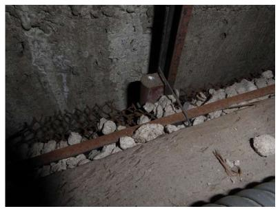
Figure 3: View looking down toward rear of fresco showing metal furring with wood nailer and attachment
