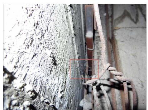
${\it View behind Fresco~3 from~above.~Note~the~form~tie~used~to~attach~the~vertical~support~to~the~wall.}$
