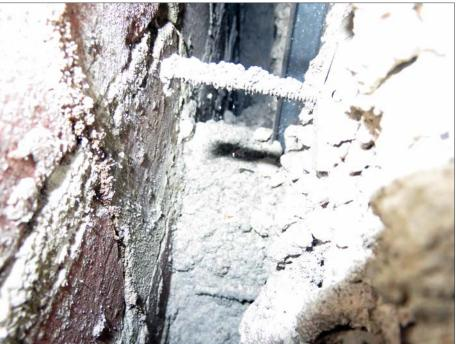
Probe 5, looking to the right and slightly down. Note the wad of mortar in the void at the furring channel. The toggle bolts are part of the handrail installation.
