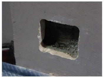
Figure 4: Decorate plaster pilaster
