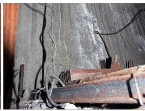
Ceiling above Fresco 7. Note the salts on the concrete from moisture infiltration and the use of the concrete form tie to hang the black iron support of the ceiling.
