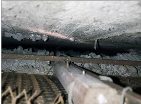
View behind Fresco 3 from above. Note the small void space and horizontal channel wire tied to the vertical furring channel. Photo by Tuan and Robinson.
