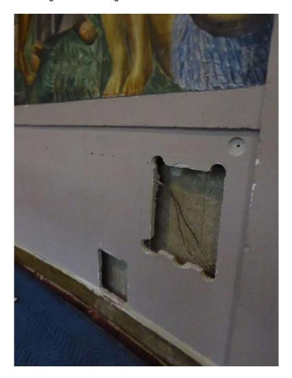
Figure 1: two access panels were removed to investigate construction and attachment of fresco wall
