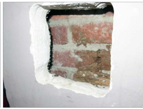
Probe 6. Note the wood block in the lower portion of the opening.
