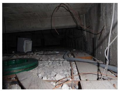
Figure 2: Image looking across plenum space above fresco wall, showing concrete rear wall, ceiling and lathe and plaster soffit.
