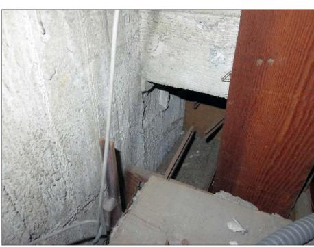
Pilaster between Frescos 3 and 4 from above. Note the board nailed to the concrete and supported furring channels of the ceiling.
