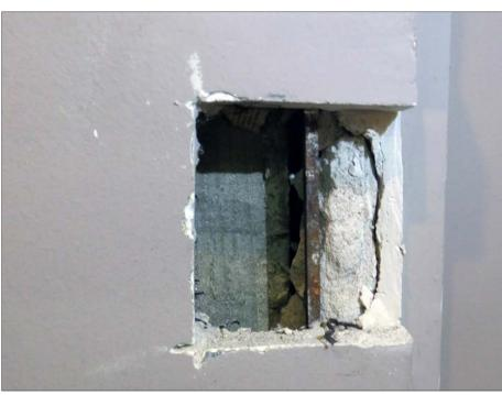
Probe 3. Note the black iron furring channel in the corner. The void space here was not filled with plaster debris, which is consistent with it being an area of repair.
