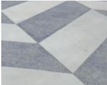
P2: cast-in-place concrete with seeded aggregate
