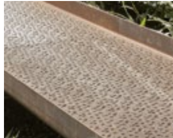
P8: slip-resistant weathered steel decking at rain garden elevated walkway
