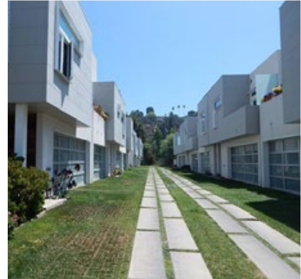
Figure 5.17-2: Permeable and vehicular rated paving is used to maximize pervious surface for stormwater management
