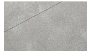
Cast-in-place concrete; medium gray w/ silica carbide and water jet finish
