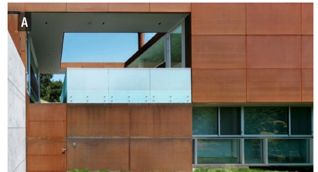
Corten steel or natural weathering steel
