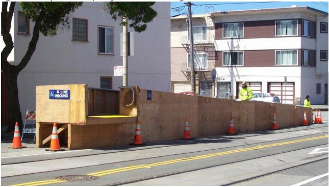
Figure 3: Example of a Temporary Accessible Boarding Island
