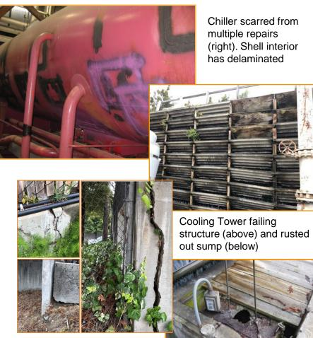
**Cooling Tower foundation** (above) structurally unstable.
