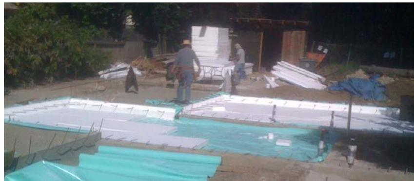
without the radiant heat activated. In addition to improving comfort, slab insulation greatly improves the home's energy balance. Slab insulation can never be retrofit, so insulating properly was important. Four-inch thick EPS sheets facilitate installation since they are less breakable than thinner sheets commonly used. Further, scraps of this thick material were used to insulate headers and wall cavities.
