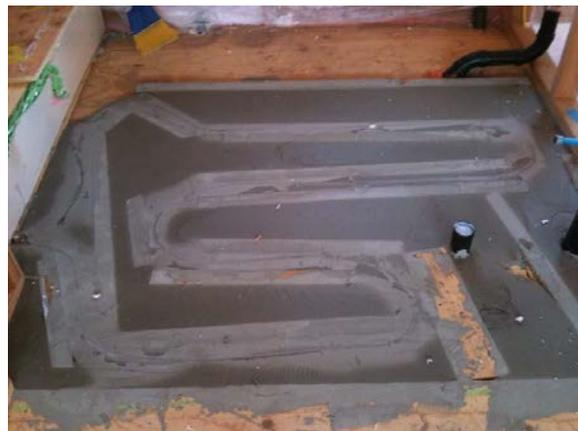
A conventional slab with tubing everywhere, running at full output, would be barely warm enough to feel, because so little heat is needed to maintain a warm room temperature.
