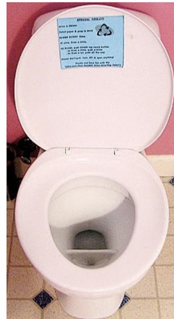
How It Works - The user simply urinates in the front drain and defecates sitting back. The drains are located so that no additional effort is needed. A dual-flush flush button features two parts: one to flush urine and one to flush solids. Each
