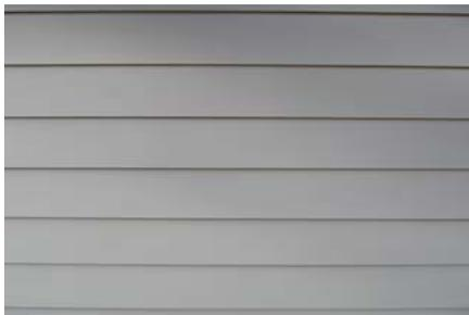
Hardie Plank is a wood fiber and cement composite material we've used for siding. It is extremely durable and dimensionally stable. The planks will last longer and have less environmental impact than other plank sidings.
