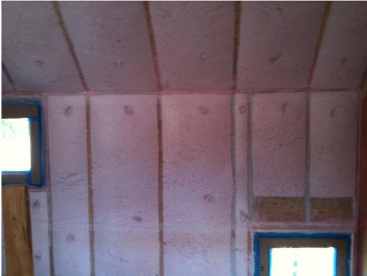
Since wood conducts heat much faster than insulation, reducing wood in the walls saves heating and cooling energy. In this house, 2x8 studs (7-1/4") are "balloon framed" over two stories, running from slab to roof, to reduce joints and connections at the intermediate floor. This also makes the house stronger against wind and earthquakes. We are looking for a student to determine if the 2x8 wood use 1) Reduces overall lumber use and 2) Given that a 2x8 requires a larger tree
